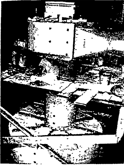
11 Early steps in applying the block insulation to cyclone separators
