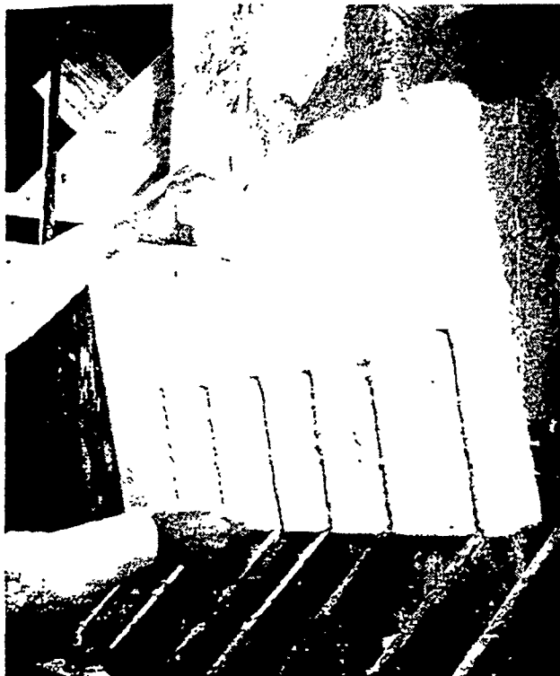
20 Specially notched block being applied to the expansion joint in the insulation surrounding the main steam lines
