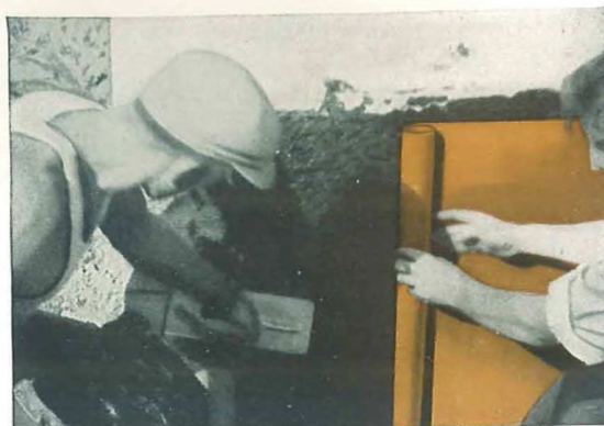
Applied with suitable mastic, this pure copper weighing 2 ounces per square foot is being securely bonded to the outside of foundation wall. Permanent damp-proofing!
