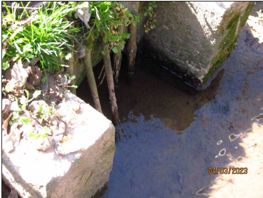
Photograph 16. (IMG_0103) View of Outfall 001 at the receiving water.
