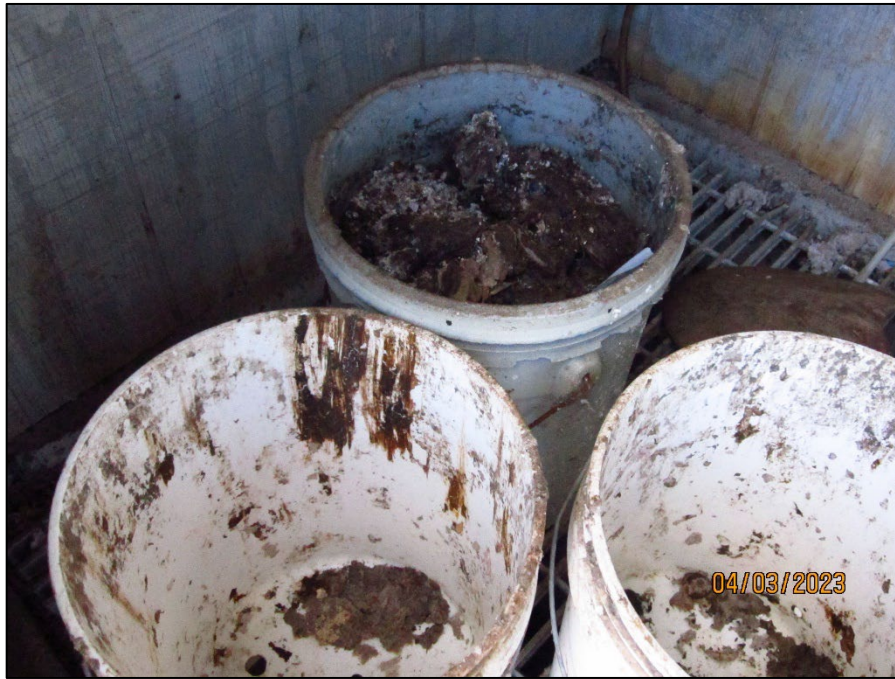
Photograph 5. (IMG_0033) View of solids stored in buckets in the headworks/influent station.
