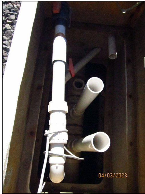
Photograph 11. (IMG_0065) View inside CCC #2
