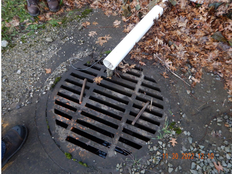
Photo 2. (DSCN5202) Plastic pipe connected to multiple roof drains on the north side of the warehouse. Stormwater was flowing from this pipe into a nearby storm drain on 11/30/2022. Sample SP-9 was taken at this location.
