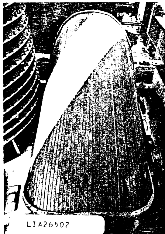
Plan view of cantilevered, doubly curved roof.
