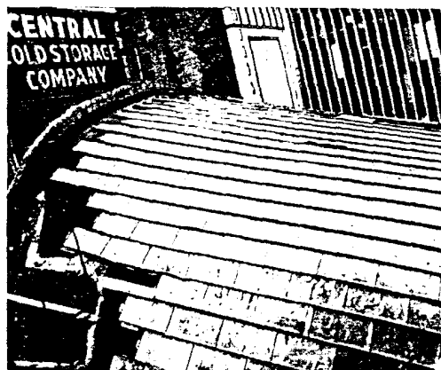
Standing seams on roof on 2 foot centers. Flat lock seams join 4 foot long panels in a staggered pattern.
