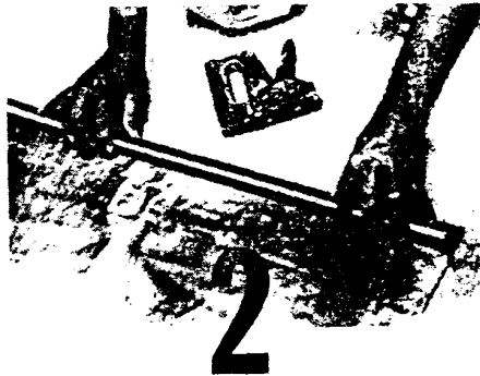
This sheet of lead, and light batten strip . . .
