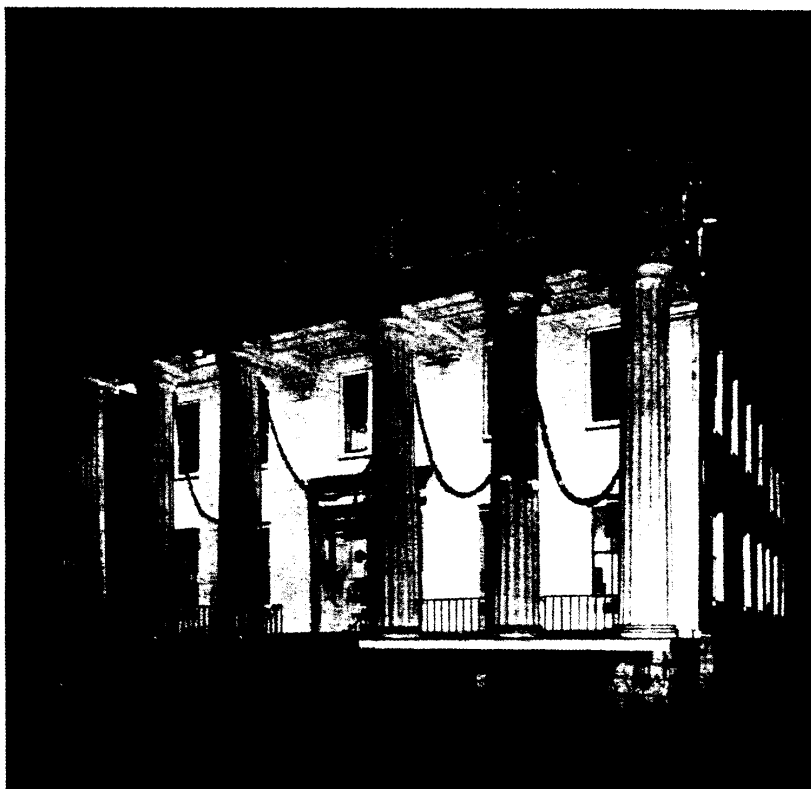
Although the main focus of attention is now on defense construction, the proper maintenance and construction of our civic and other peace-time buildings should not be neglected. The Department of Education Building, Schenectady, N. Y., is an example of good maintenance practice, with white lead, which should be continued for all types of construction during these critical times. (Article on Page 5)
