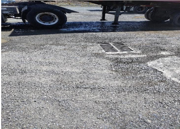
IMG 8864 -Storm inlet in north of CommUseArea 1. IMG 6541 -Storm inlet midway in CommUseArea 1. The storm inlet is not protected from the influent of The stormwater basins are aligned in series from east gravel, sediment and trash carried by stormwater runoff flows to west across the referenced area.
