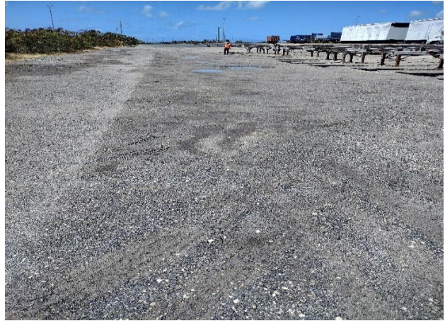
IMG 5595 -Unpaved south area of CommUserArea 1. Grade allows stormwater flow from east to west.
