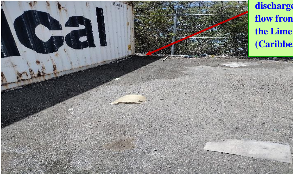
IMG 1793- Discharge point where storm water from the rear yard area of the maintenance shed reaches the a point along the western fence line of the Facility, and drains into Lime Tree Bay.
