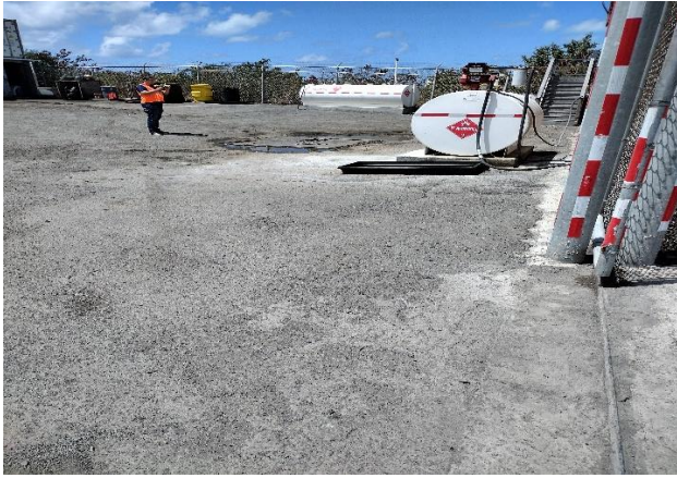
IMG 5366 -Fueling terminal unit within fenced area of Tropical's maintenance shed. Yard surface slopes toward large stormwater catch basin.
