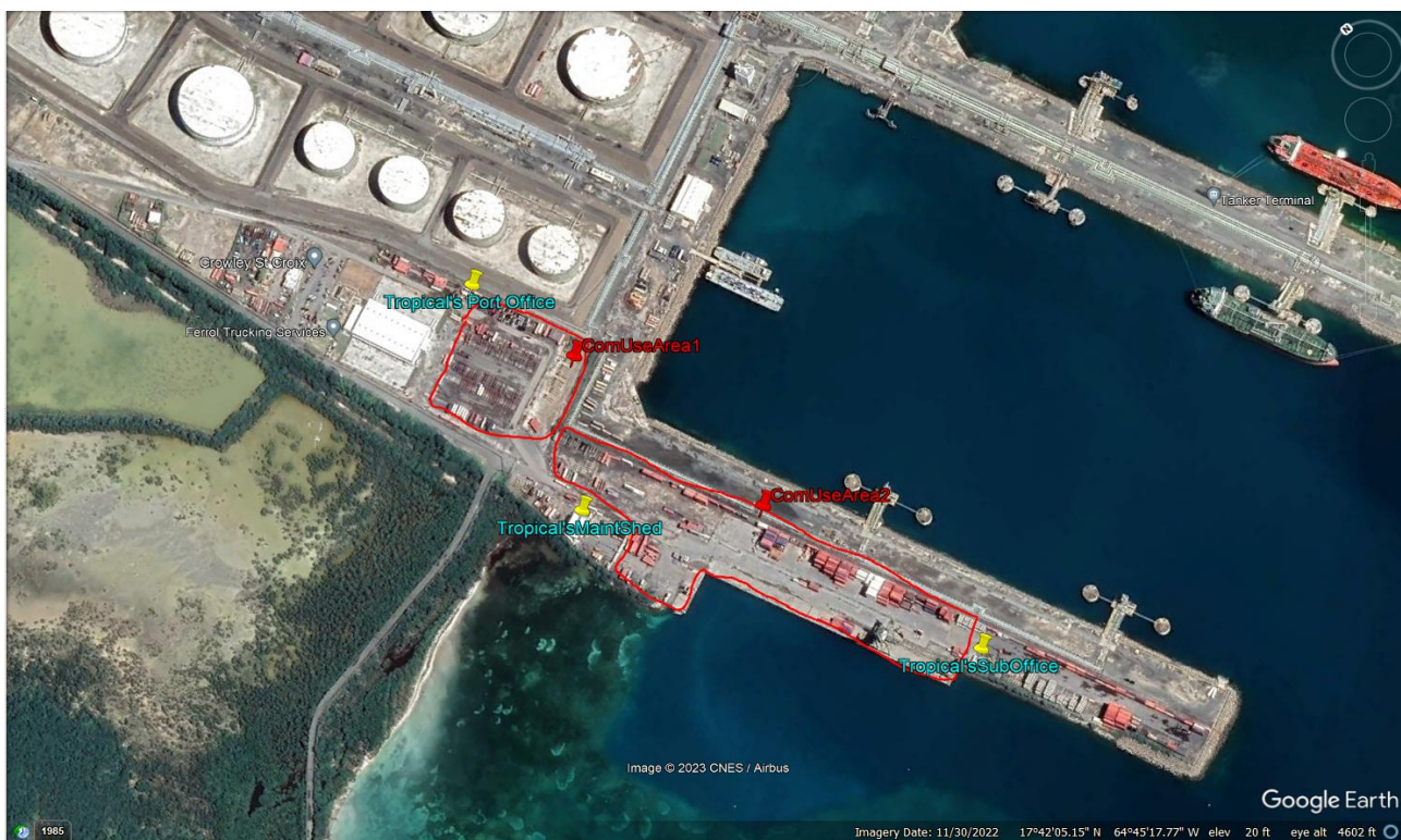
Figure 1 Tropical’s Container Port Marine Cargo Terminal, Christiansted, St. Croix, VI
