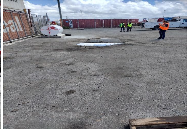
IMG 5320 -Sloped yard surface towards large stormwater catch basin within the fenced area of the maintenance shed. Basin not within a containment.
