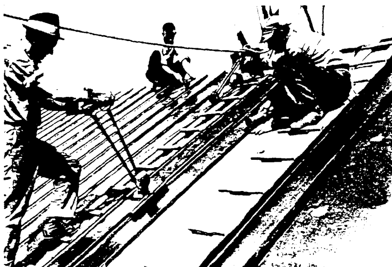
Workmen installing a standing seam terne plate roof.
