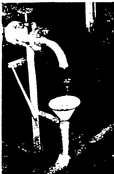
The flow of liquid alum through lead pipes from the storage tank to the water tank is controlled by a pinchcock.
