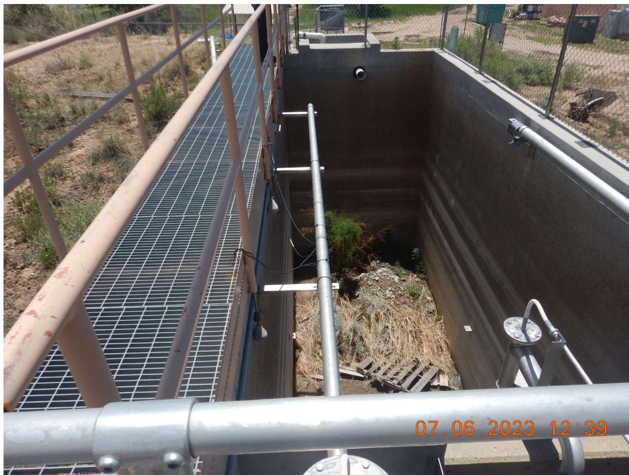
An overall view of the inside of the decommissioned Towa WWTP treatment process basins. (DSCN 2561). Photographed by D. Esparza.
