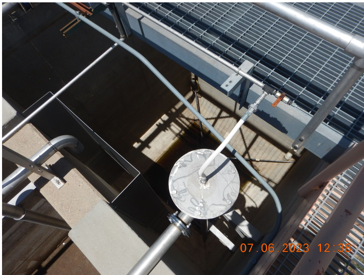
Another view of the inside of the decommissioned Towa WWTP treatment process basins. (DSCN 2560). Photographed by D. Esparza.
