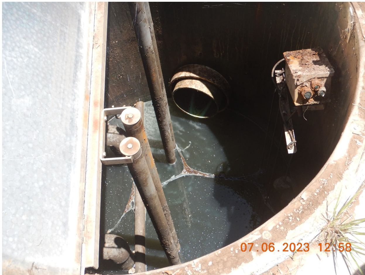
View of the inside of the decommissioned WWTP wet well. Note: the standing water was a result of a previous rain event. (DSCN 2567). Photographed by D. Esparza.
