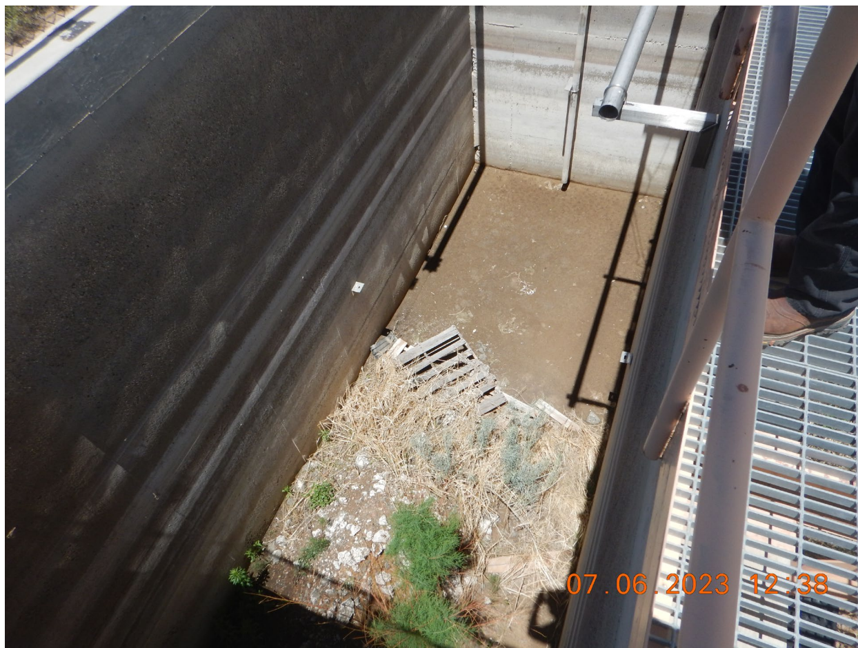
Picture of the inside of the decommissioned Towa WWTP treatment process basins. (DSCN 2559). Photographed by D. Esparza.
