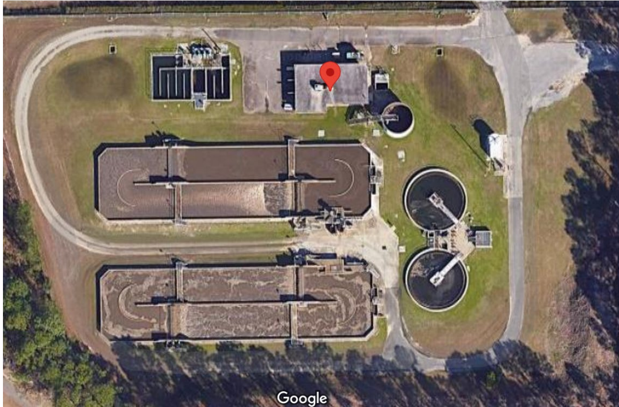
Figure 1 – Facility Aerial View
