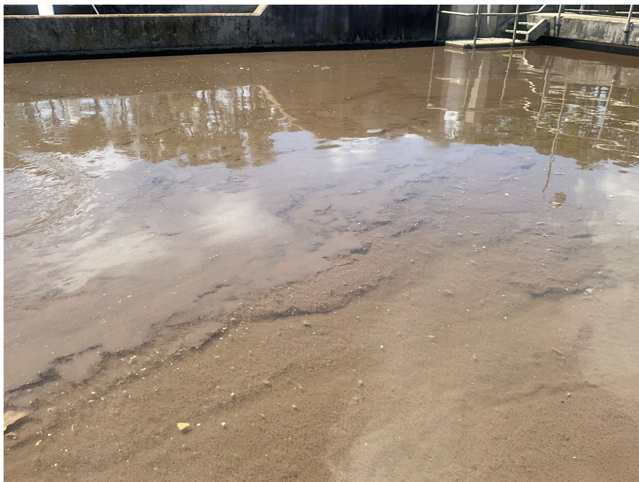
Figure 2 – Grit presence in Oxidation Ditch
