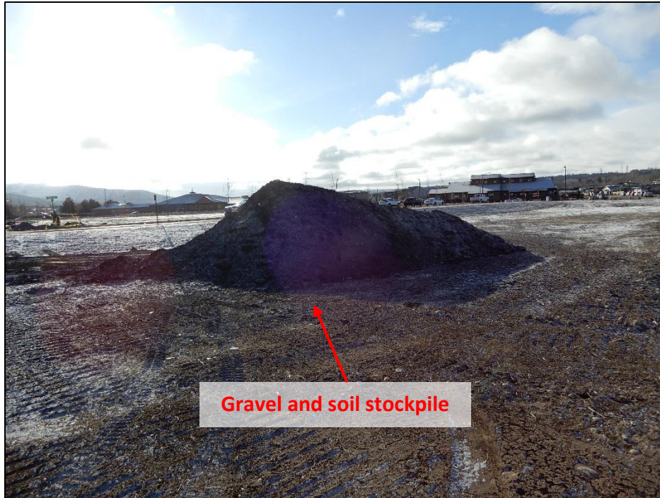
Photograph 5. View, facing east, of an unstabilized gravel and soil stockpile. It was noted that fiber rolls were installed downgradient of the stockpile along Warm Springs Creek that provided perimeter protection.
