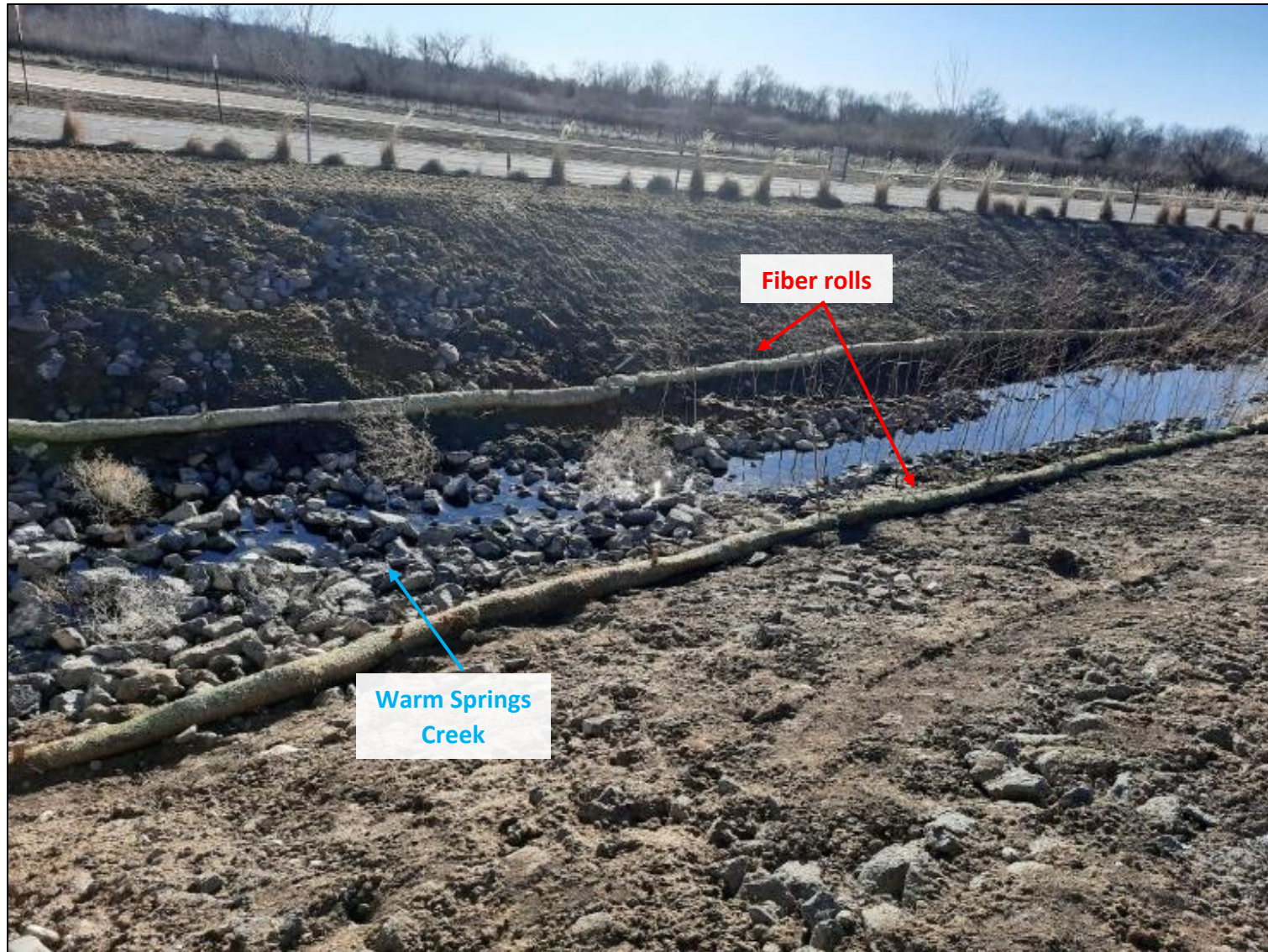
Exhibit 3. View, facing southwest, of Warm Springs Creek, west of East Millbrook Way. The fiber rolls were moved downgradient of the hydro seeded area along the creek. The image was sent to the Inspection Team from Kyle Terrell on 3/2/2021.
