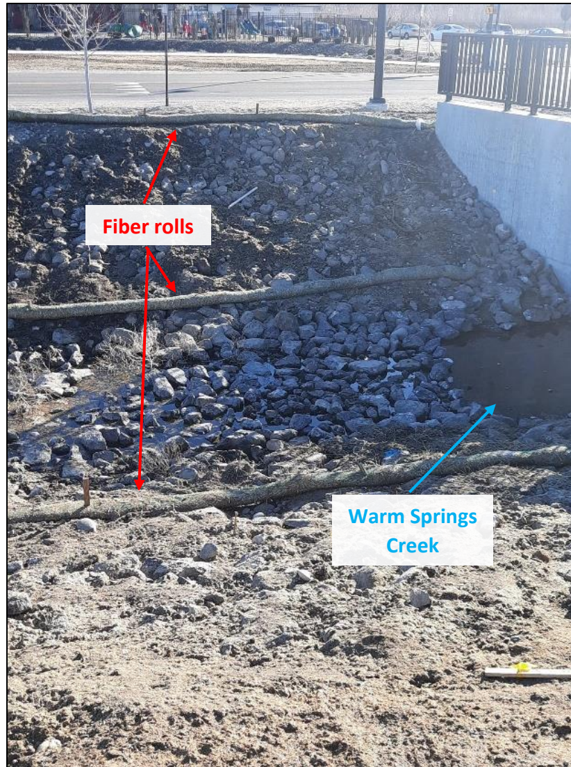
Exhibit 5. View, facing south, of Warm Springs Creek east of East Millbrook Way. Fiber rolls, as stated by Kyle Terrell, had been added downgradient of the hydro seeded area along the creek. The location shown is east of the location shown by Exhibits 3 and 4 . The image was sent to the Inspection Team from Kyle Terrell on 3/2/2021.
