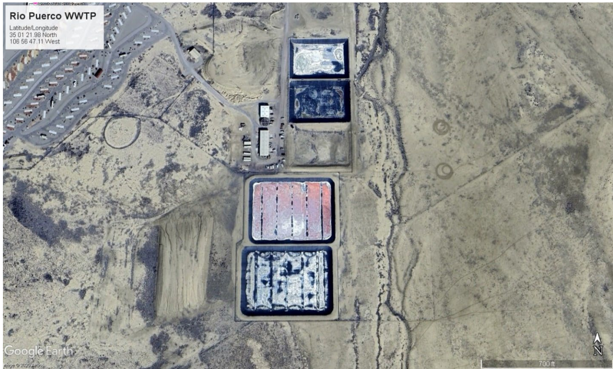
Aerial Image #1: Overall view of the Laguna Development Corporation-Rio Puerco Wastewater Treatment Plant Location. Aerial from Google Earth Maps
