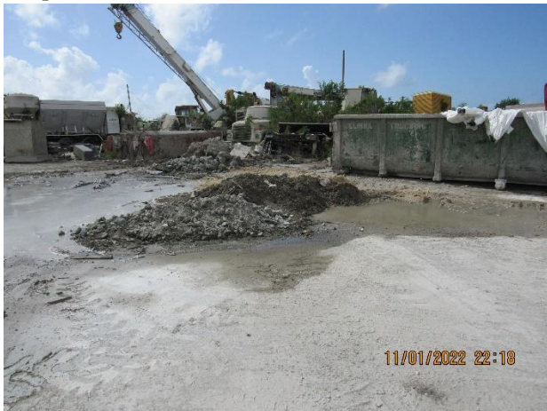
IMG 773 -Edge of the pond where spent concrete to a berm. The berm ineffective because a dry-weather flow drained from the pond. and out of the Facility. wastewater).
