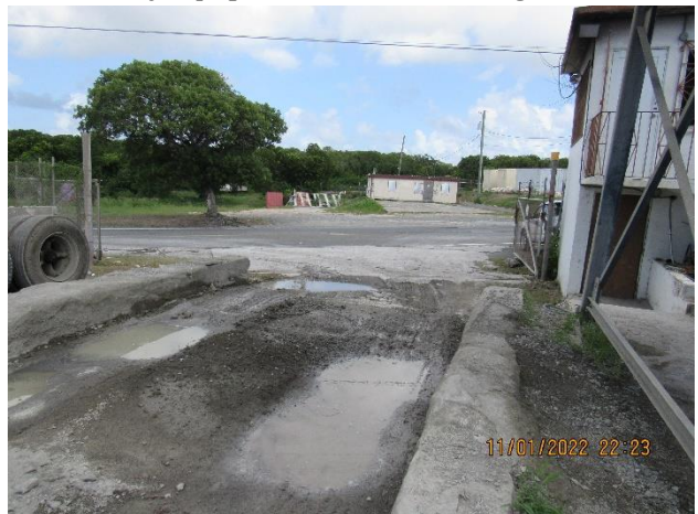
IMG 780 -Close-up of the ready-mixed concrete loading bay, inclined down towards the public road.
