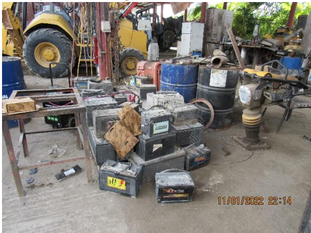
IMG 771- Accummulation of spent auto batteries situated on floor of maintenance shed in potentially managed under incompatible conditions.
