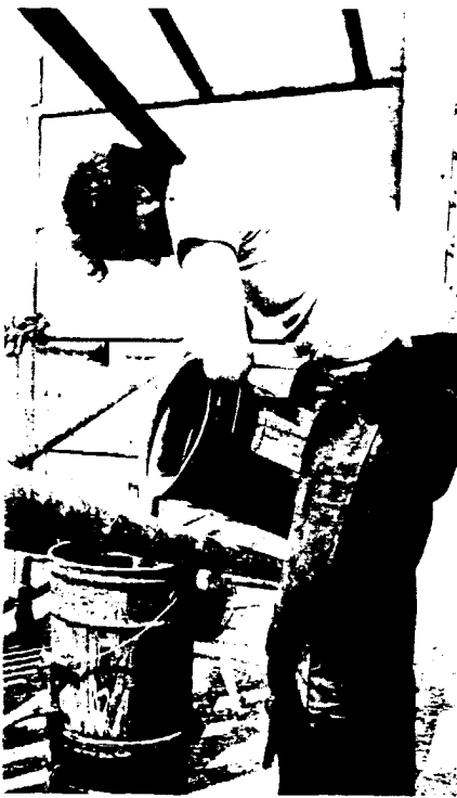
Red lead paint poured into can travels through tube which extends down through cutouts in bridge deck and flows into portable "dam" which surrounds bottom 3 1/2 ft. of the bridge cable.
