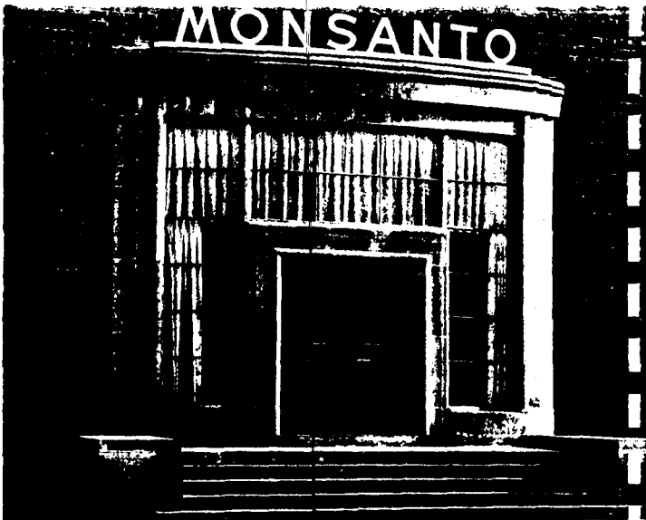
Entrance to office and laboratory building at Trenton, Michigan, plant.
