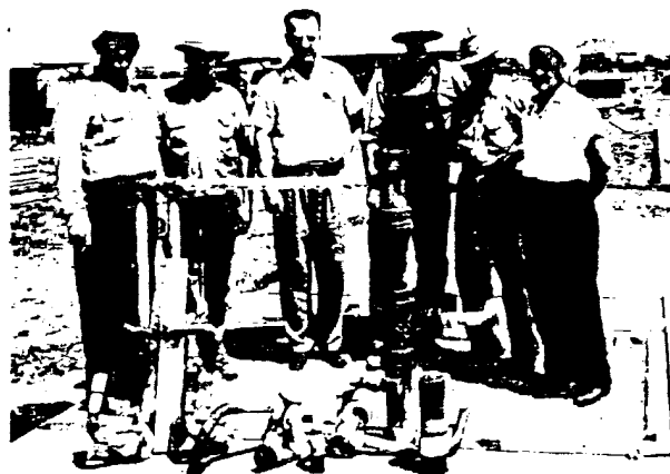
Plumbing Inspector Simms, left, plumbing contractor Richardson, center, with journeymen plumbers looking over lead fittings to be installed in housing project outside of city limits in compliance with Port Arthur plumbing code
