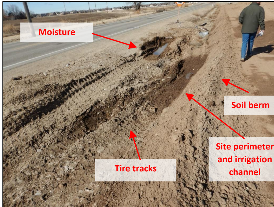
Photograph 9. View, facing northwest, of the irrigation channel on the northwestern perimeter of the Site along South Eagle Road. Note the moisture and the tire tracks in the irrigation channel and the soil berm.
