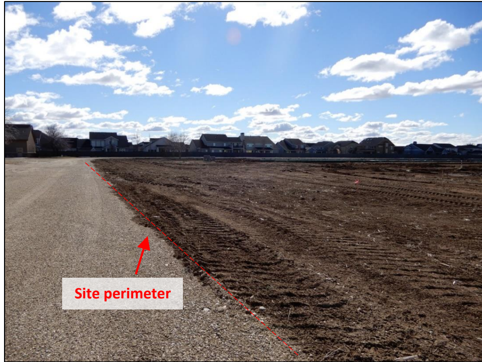
Photograph 7. View, facing south, of the southeast perimeter of the Site (photograph taken from off site). Note the lack of perimeter controls.
