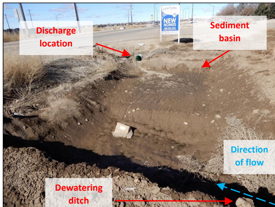
Photograph 6. Another view, facing north, of the sediment basin located on the northwest perimeter of the Site. Note the dewatering ditch leading to the basin, signs of previous containment of water, and the discharge point from the northwest perimeter.
