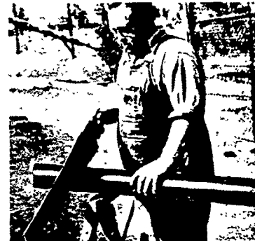
Pipe can be easily cut on location with ordinary hand saw.
