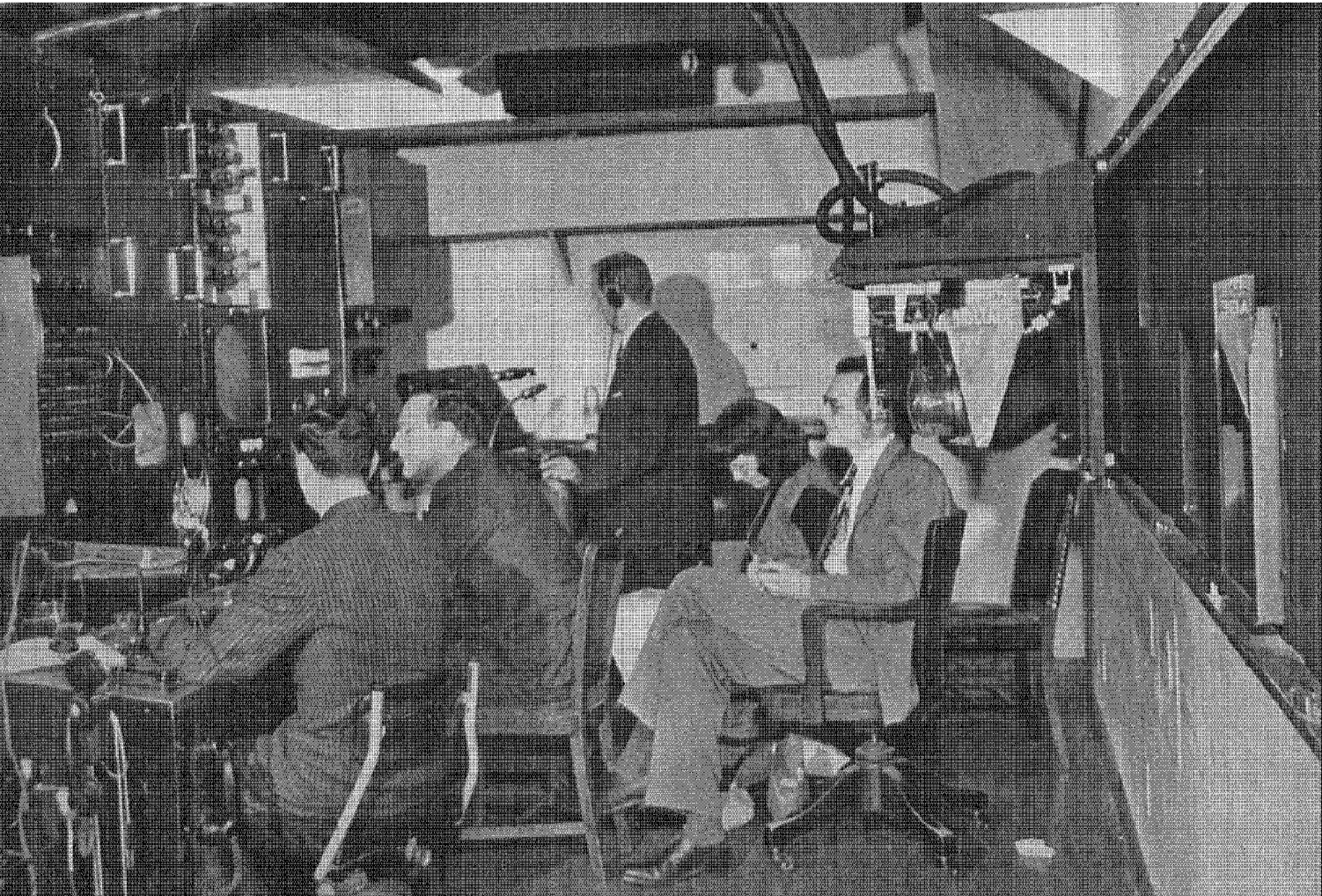
● In the National Broadcasting Company's film control studio, engineers preview the film as it goes on the air four hours after the ceremony in Washington.
