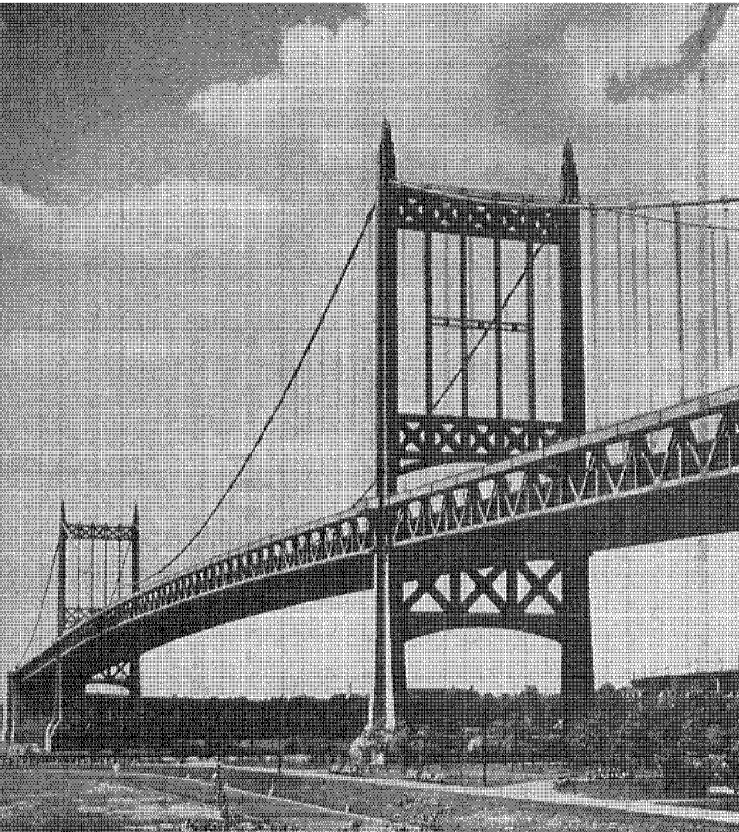
"Dulux" protects giant East River Crossing of the Tri-borough Bridge against industrial fumes.
