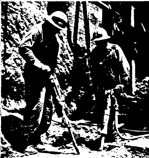
Diesel-powered pumps supply compressed air for "concrete busters" used in excavating remnants of buildings formerly on the new skyscraper site.
