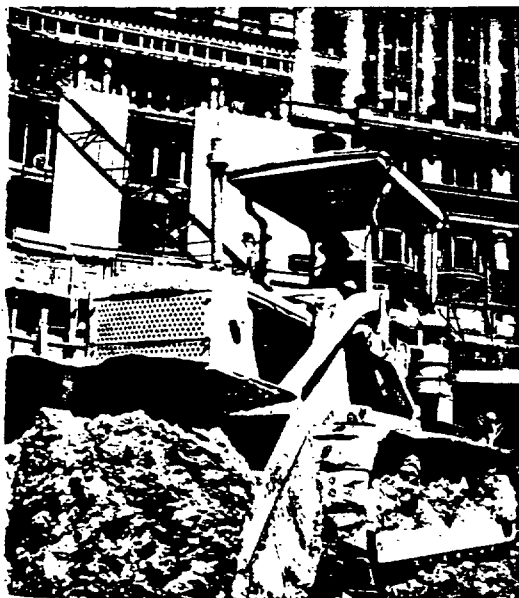
With exhaust roaring, this front-end loader fills its maw with soil and rock to be hauled away.
