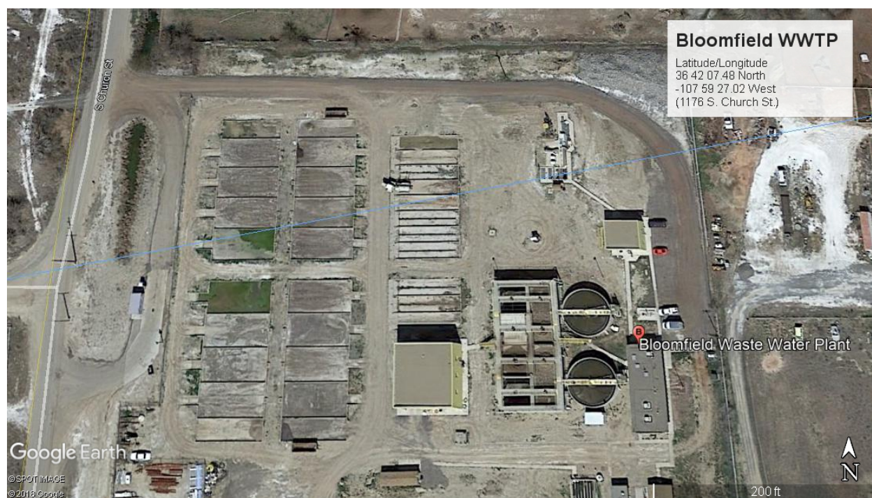
Aerial Image #1: Overall view of the City of Bloomfield Wastewater Treatment Plant. Aerial from Google Earth maps.
