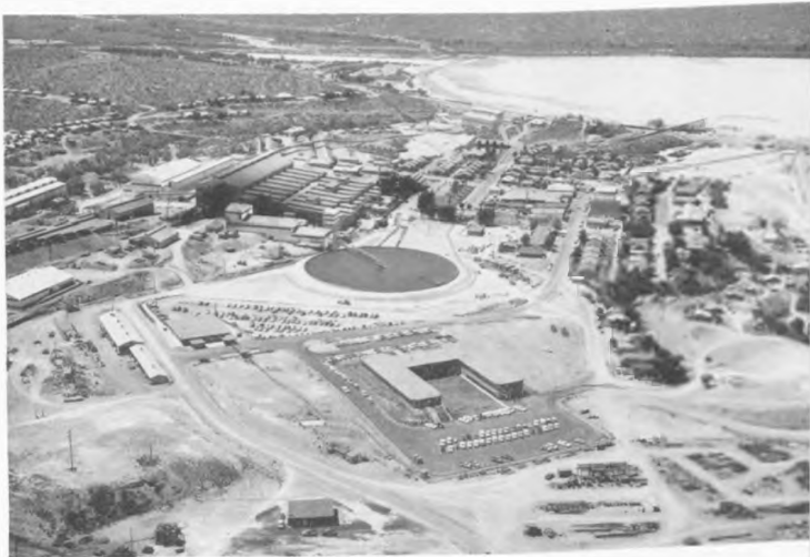
New ore crushing plants, and shops were built. The capacity of the mill was increased 50 per cent to permit handling the larger amount of ore that can be mined.
