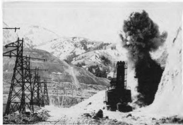
Blasting at One of Kennecott's Open Pit Mines. Large electric shovels will scoop up the loosened material into railroad cars for hauling to the mill.
