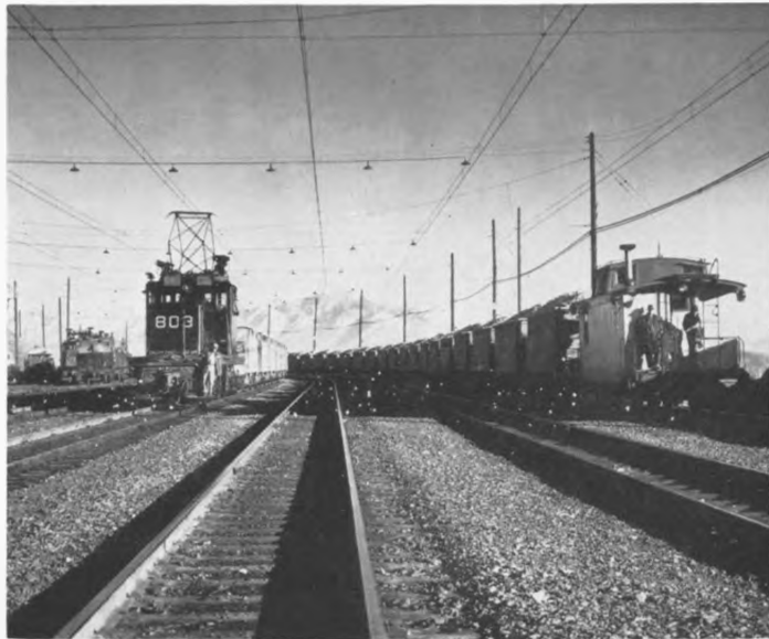
Ore Haulage from Mine to Mill. At the Utah division cars carry about 90 tons of ore each. Approximately 1,000 carloads are hauled to the mill daily.
