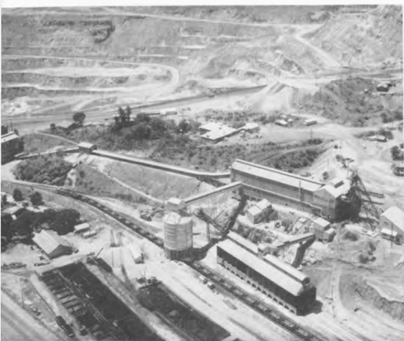
The pit was enlarged to permit expansion of mining. Additional ore storage capacity, new 100-ton ore cars, and greater belt-conveyor capacity were added.
