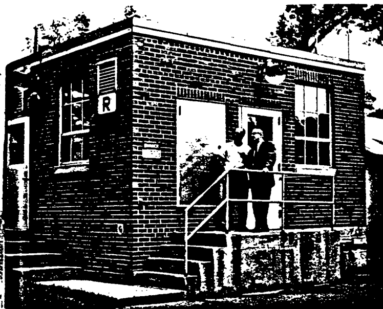
Above, on the steps of the fleet-blend installation, Wes Price and Reg Broquet, right, are discussing a problem on a tank truck delivery.
