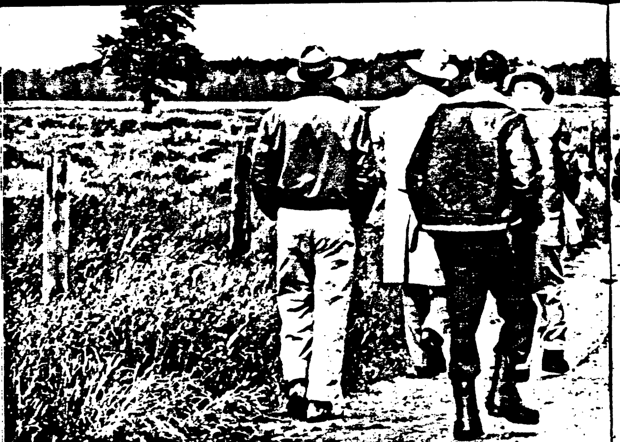
Above, Ethyl and Oliver engineers follow their brain-child down a road at the 1954 field trials where the OX-121 was first put through its paces. With the successful completion of these tests, any fears that the gasoline tractor might have outlived its
