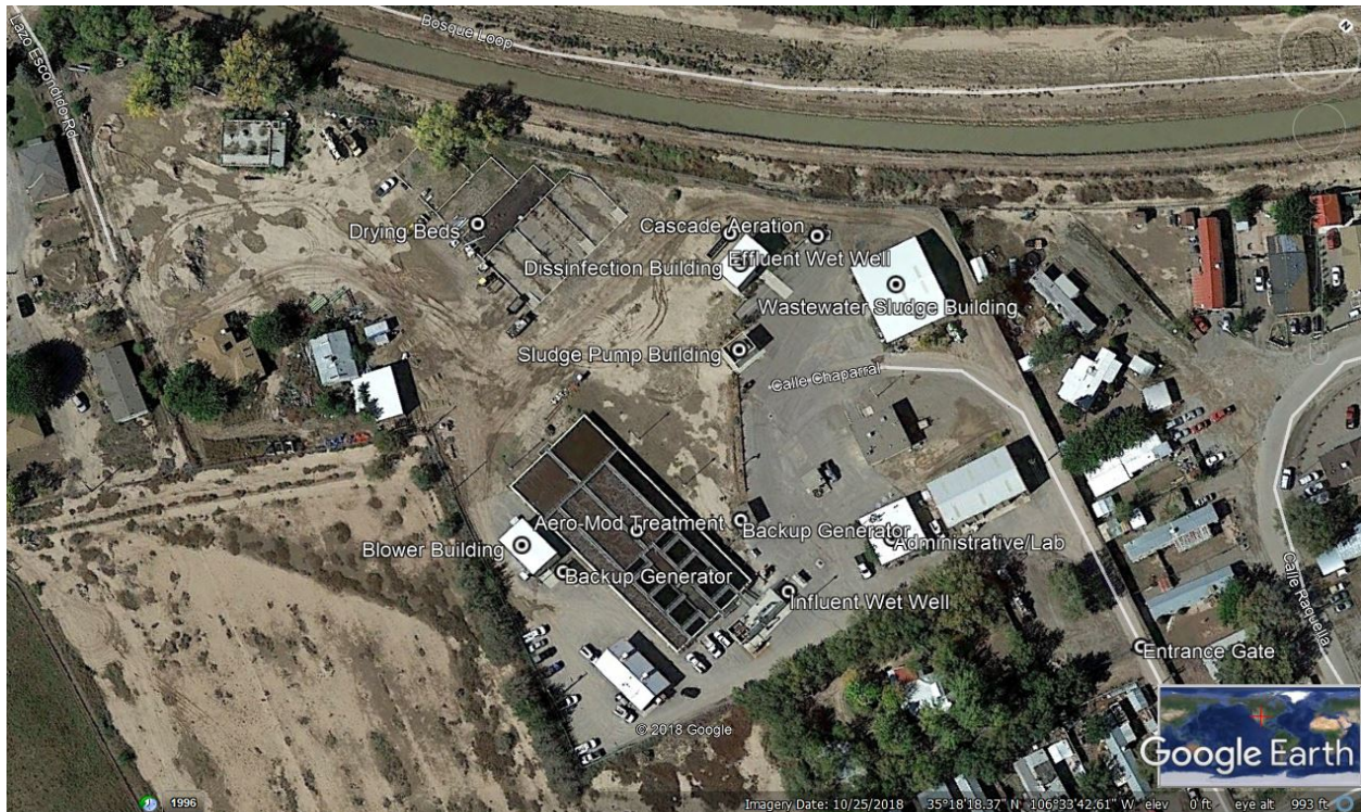
Aerial Image #1- Overall view of the Town of Bernalillo Wastewater Treatment Plant. Aerial from Google Earth.
