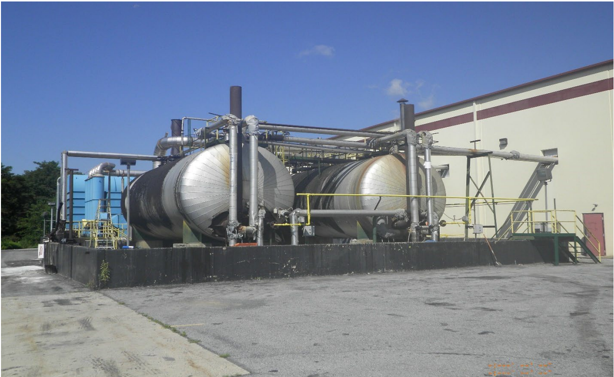
12. Two Heated Hot Asphalt Tanks – Warrior Roofing – 7/19/22
