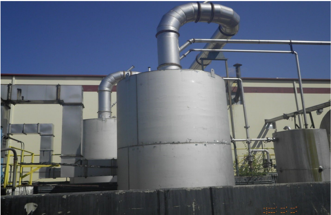
14. Oil Knockout Tank – Warrior Roofing – 7/19/22
