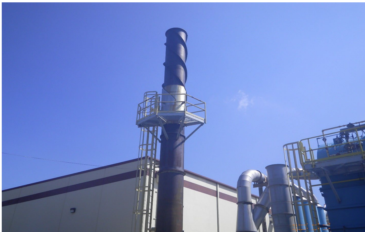
16. Regenerative Thermal Oxidizer Stack – Warrior Roofing – 7/19/22
