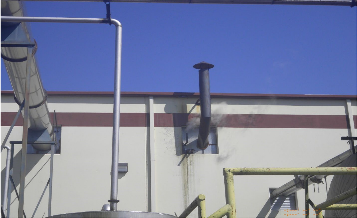
13. Steam Generator Stack – Warrior Roofing – 7/19/22
