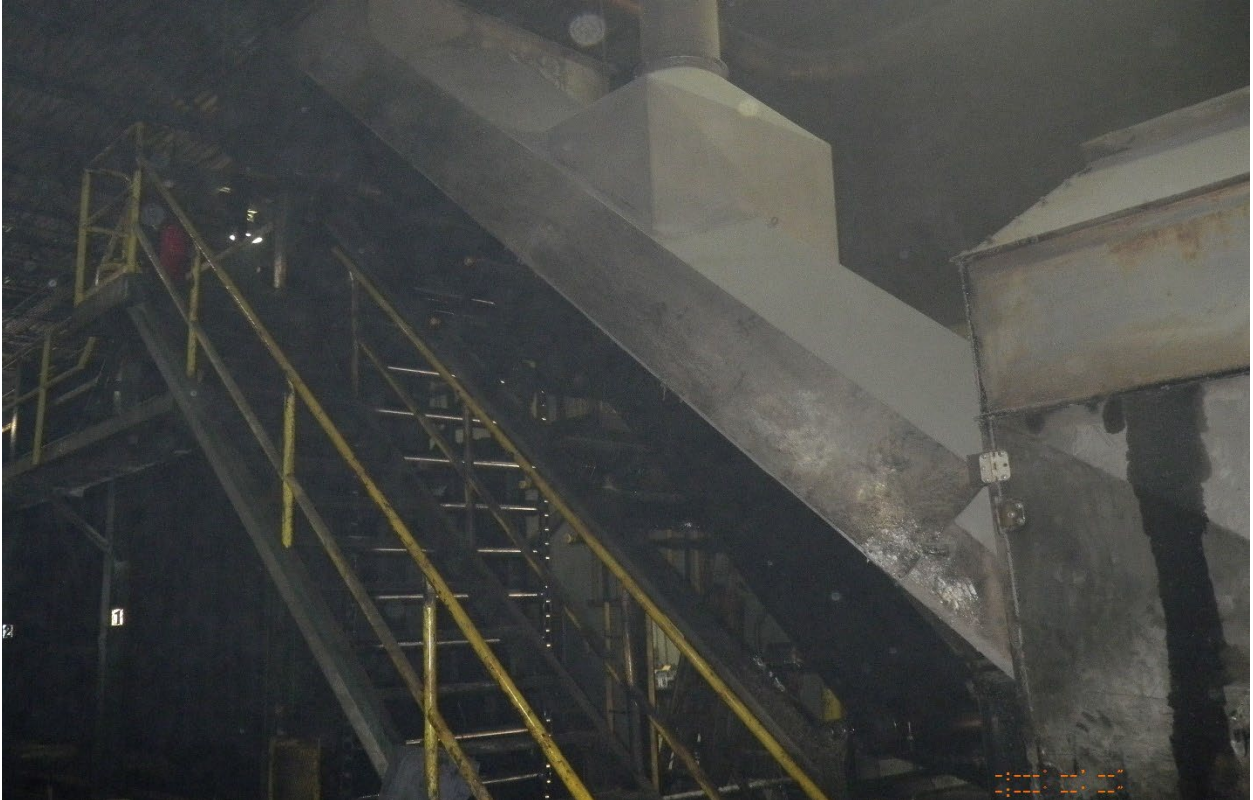
6. Saturated Paper Incline Ramp Line 1 – Warrior Roofing – 7/19/22
