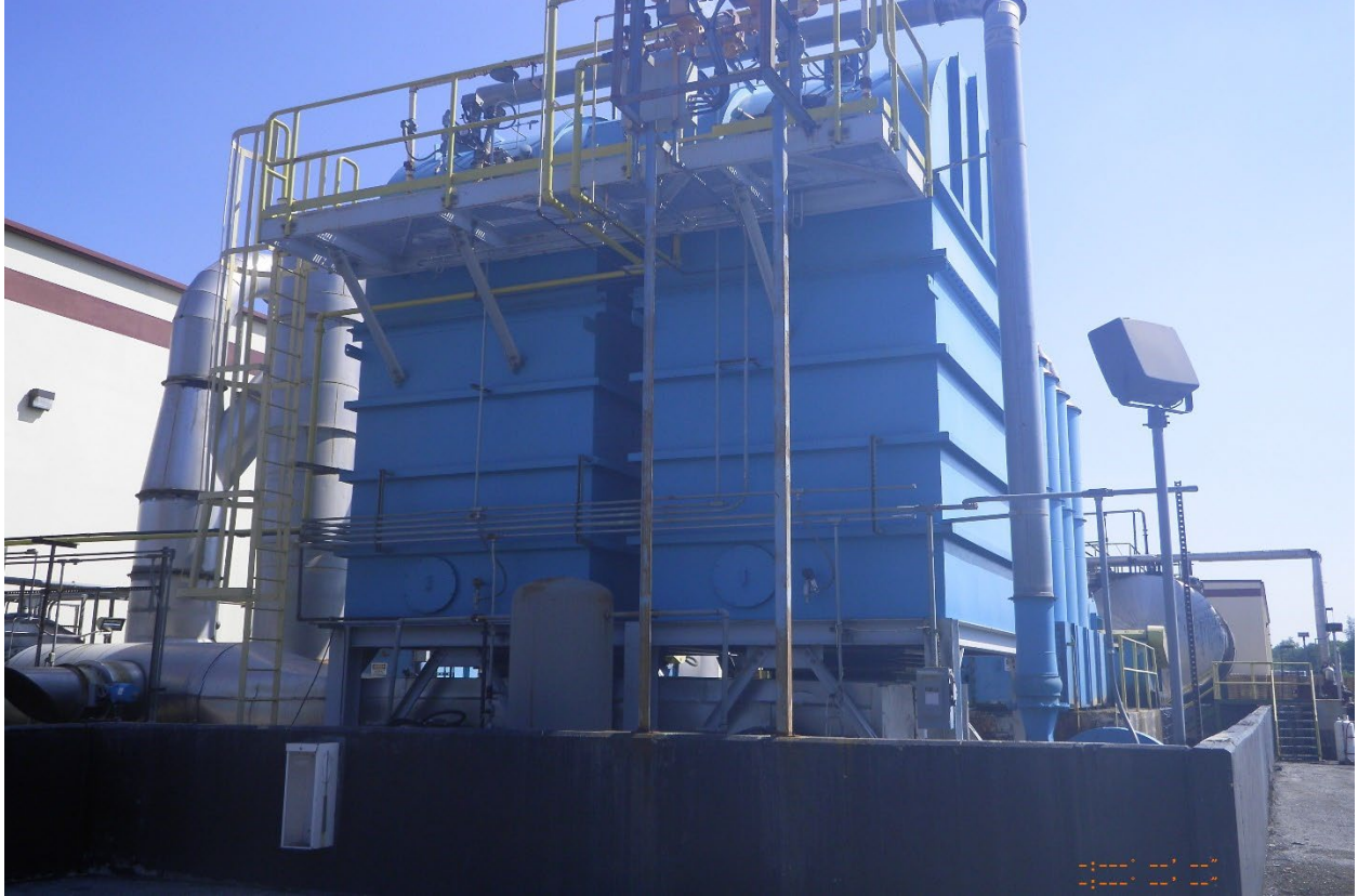
17. Regenerative Thermal Oxidizer Combustion Chambers – Warrior Roofing – 7/19/22
