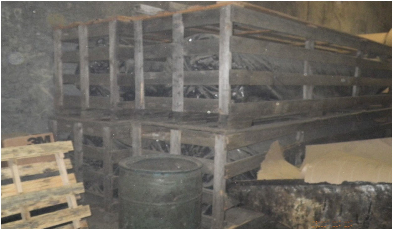
18. Extra CECO Air Filters – Warrior Roofing – 7/19/22
