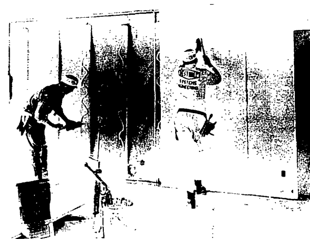
Completion of partition
