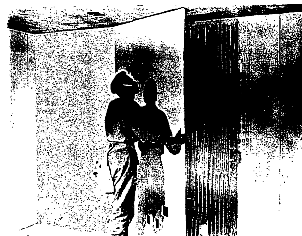
Face layer being laminated
