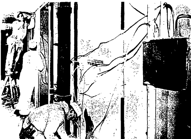
Electrical work roughed in, ready for 1" coreboard
