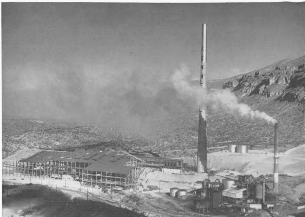
The new smelter under construction for the Ray Mines Division with the completed 600-foot stack. L-P-F plant is in right foreground.
