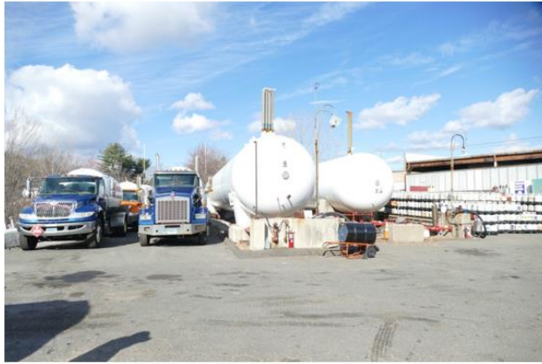
30,000-gallon and 60,000-gallon tanks of propane, filled by trucks. Not in compliance with industry standards of care (NFPA 58).
