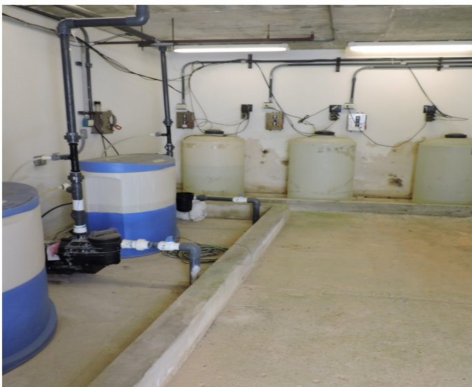
Picture 146 - UPR SWIMMING POOL AREA - At the Swimming Pool Area, the Pulsar 4 System controls and applies chemicals as needed to the pool water, and on a routine basis, and therefore, there is not any chemical storage room at the swimming pool area .
