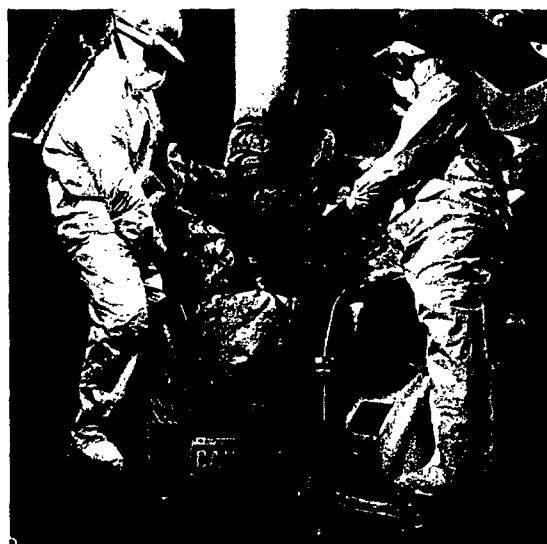
Workers removing asbestos from pipe are protected from possible harmful exposure by coveralls and hoods of Tyvek spunbonded olefin material. Use of personal protective equipment is one way to guard against the adverse health effects of asbestos fibers. (Photo courtesy of Du Pont Co.)
