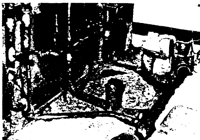
Above—Four in. lead soil line serving seven fixtures in new toilet room in Tulsa World Building in Tulsa, Okla. All fixture connections and vent branches also of lead.
