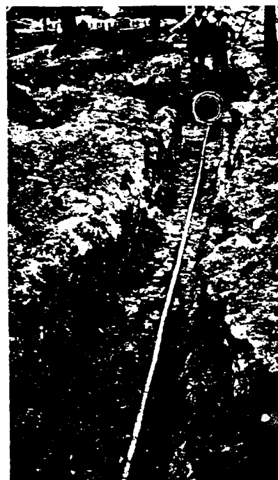
Unusually long water service installed in lead with minimum number of joints.
