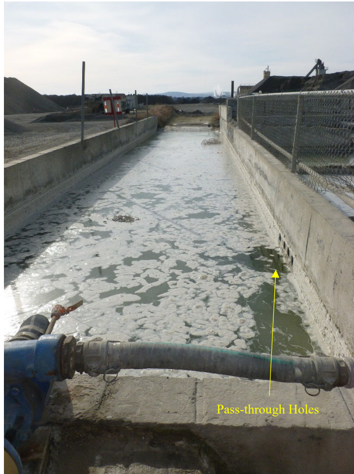
Photo 9/P1010586 – Concrete Pond
