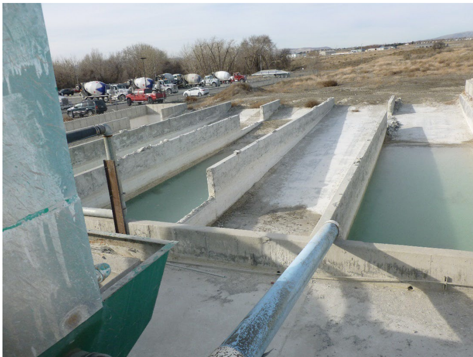
Photo 10/ P1010586 – Concrete Reclamation Water Settling Pond
