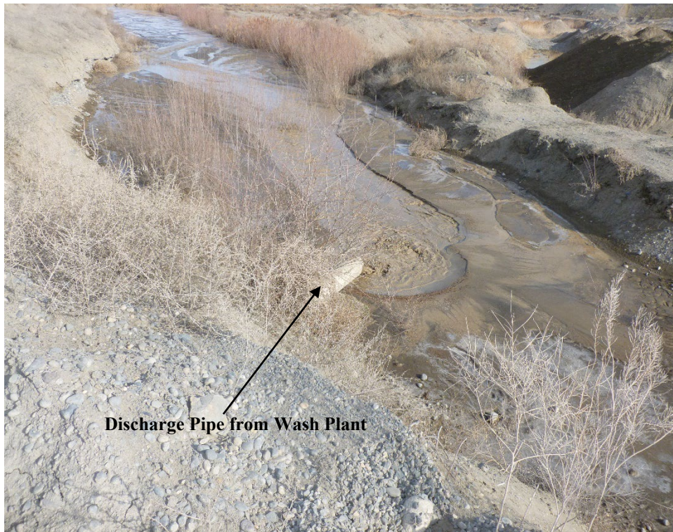
Photo 5/P1010581 – Discharge from Wash Plant, photo 1
