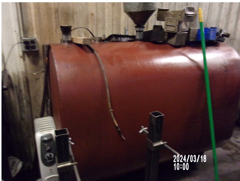
Photograph 5: Used Oil tank in the Transmission Rebuild Area.
