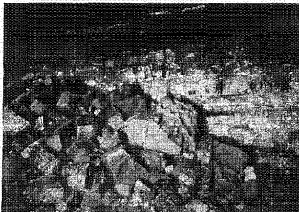
This view shows the result of a shot. Note that the coal is broken in large lumps by the blast
