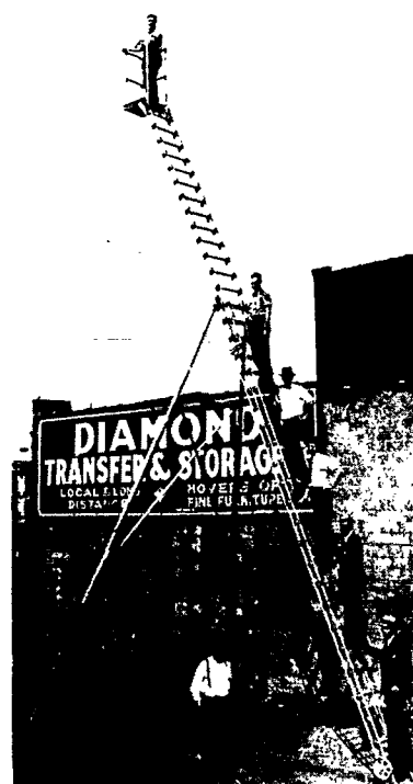
Light weight alloys make strong, serviceable ladders but they cannot compete with wood in price. This 44-foot extension ladder weighs only 172 pounds complete. The leg brace is removable.
