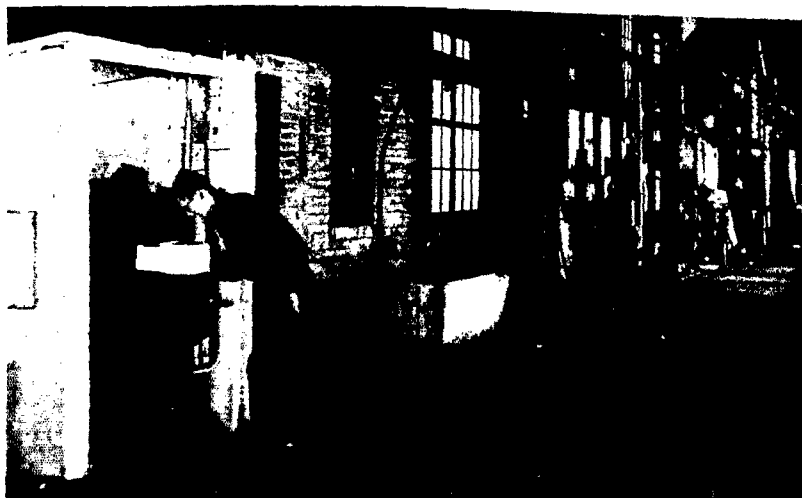
Frigidaire Corp. This fountain with a guarded jet which cannot be touched with the lips provides water at regulated temperature. Artificial cooling is usually more economical than leaving a tap running.
