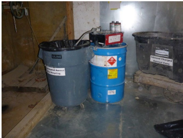
Old Pump Room - Photo 29: 55-gallon drum in the Aerosol Can Puncture Station SAA. Drum was labeled hazardous waste D001, F003, F005 waste paint related material and marked with an indication of the hazards on the product label.
