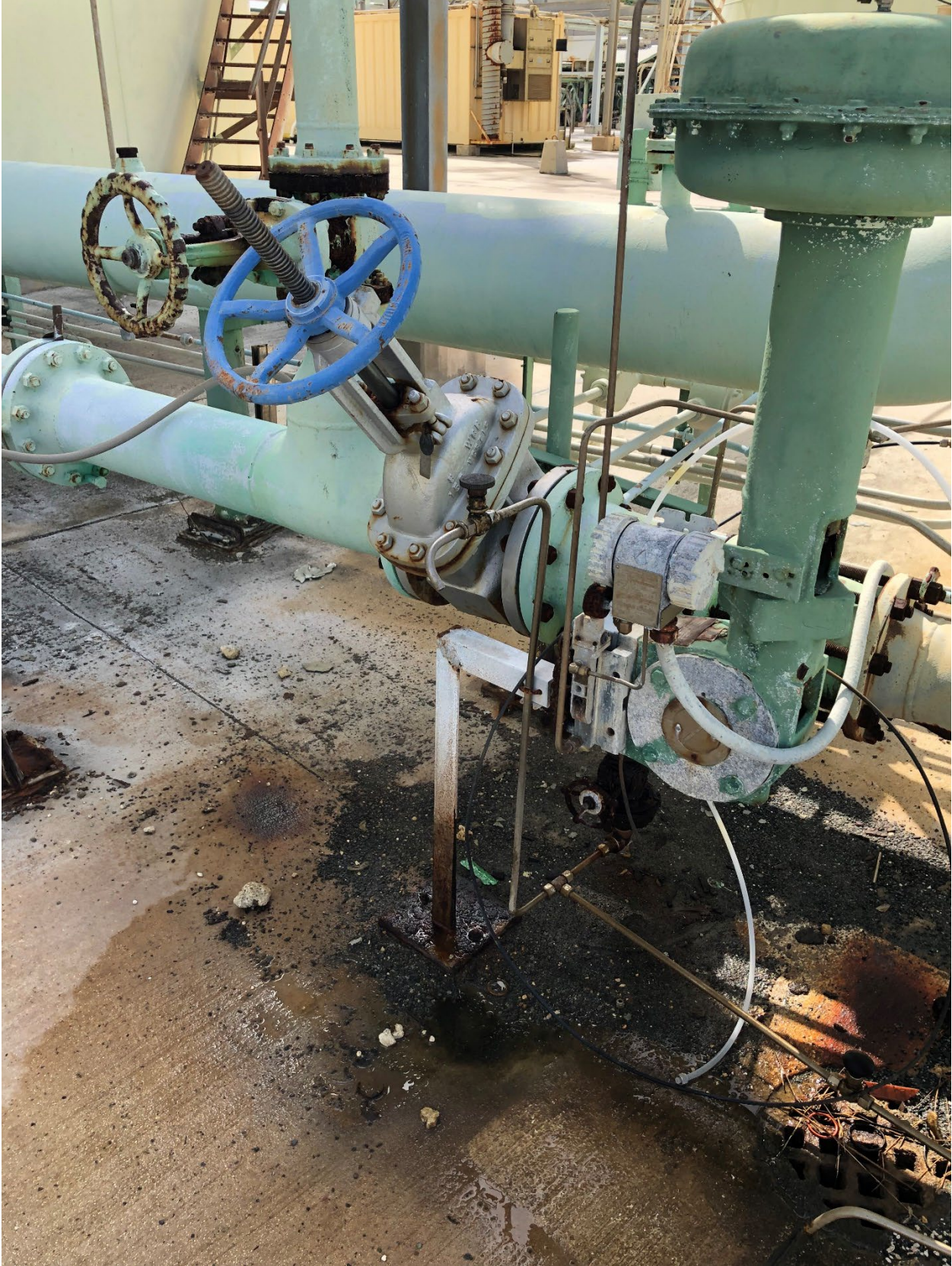
Photo #2: Sample tap for Outfall 401 where grab samples were collected.
