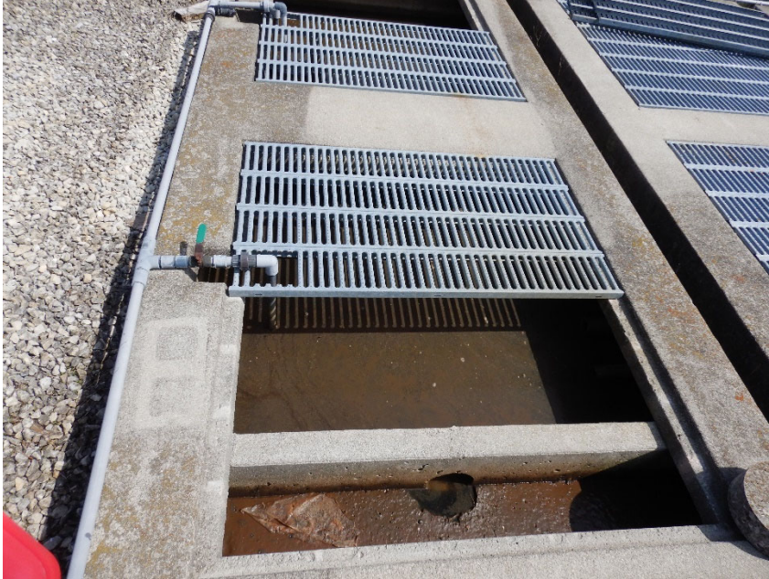
6: DSCN0765 Description: Sludge holding tank/digester Location: Wastewater treatment plant Camera Direction: down Date/Time: 4/1/2025 14:37
