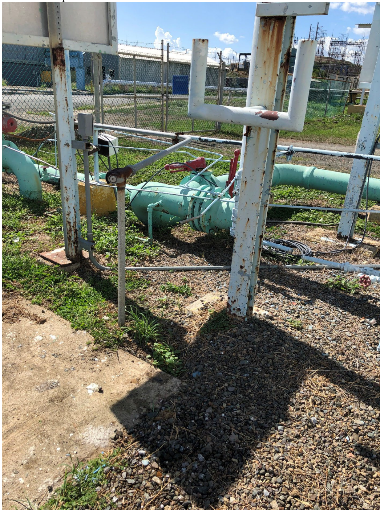
Photo #1: Sample location for Outfall 003a.
