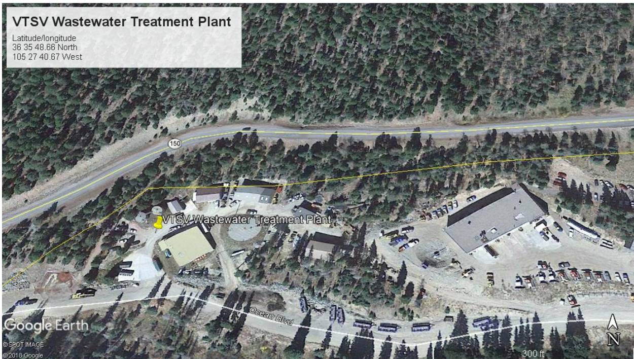
Aerial Image #1: Overall view of the Village of Taos Ski Valley's Wastewater Treatment Plant. Aerial from Google Earth maps.
