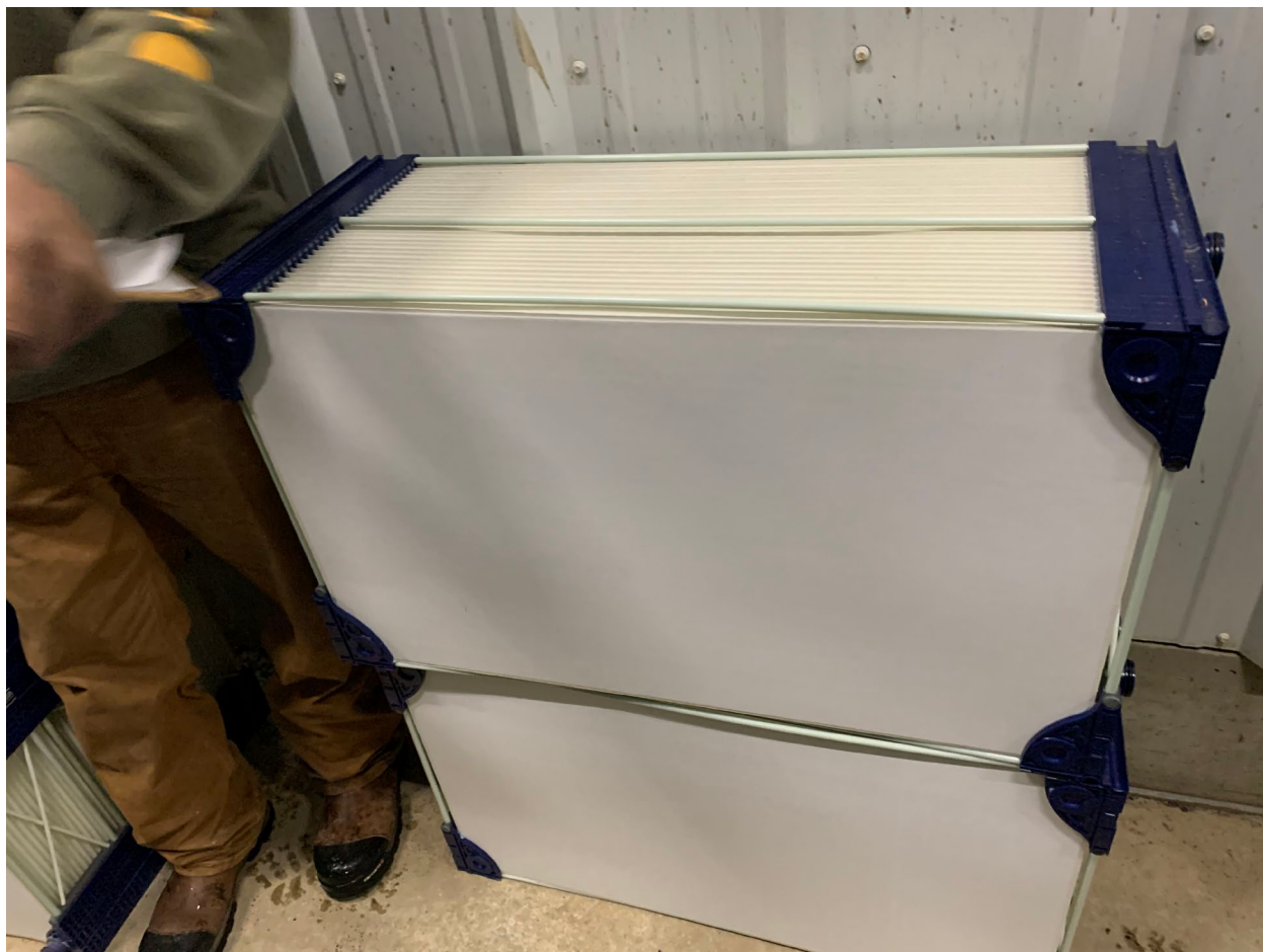
View of some of the Ovivo MBR membrane modules. (IMG_0218). (10:16 AM :01/18/2024). Photographed by D. Esparza
