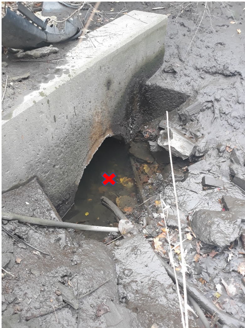
Scofield: Outfall located on the south east bank of the bridge at the north end of Scofield Avenue. Sample point is indicated by a red “x”.
