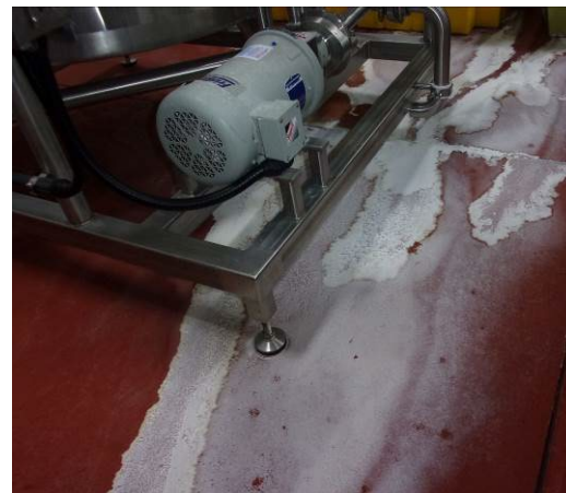
Figure 16: 10:15 AM CIP Room
