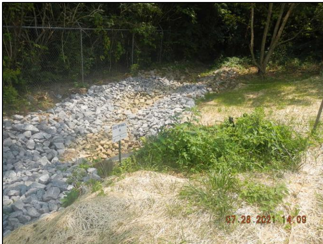
Photo 3: Outfall 004 (to Dry Run).
