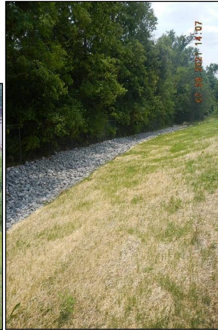
Photo 2: Remediated area upstream of Outfall 004.
