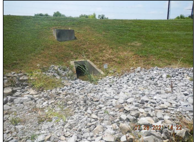
Photo 4: Outfall 003 (in detention basin).
