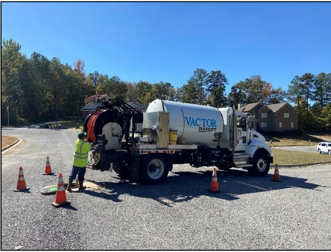
Photo 1. County jet/vac truck.
