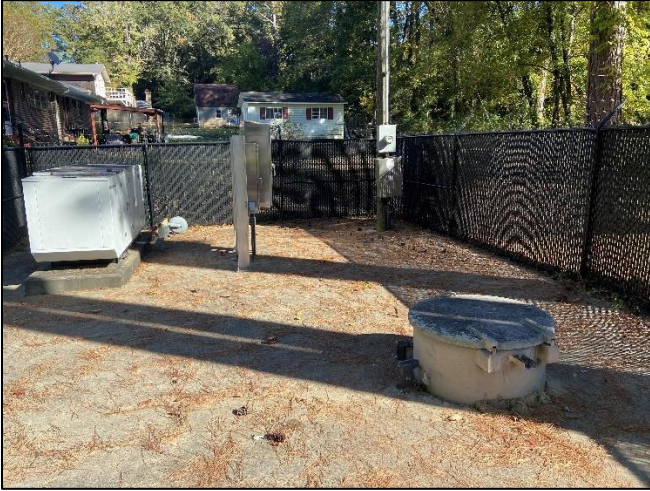
Photo 5: Walker Avenue pump station.
