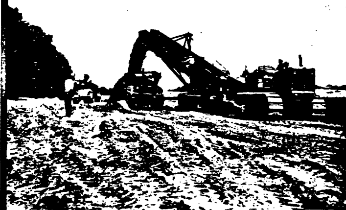
Expensive as actual construction work is, it is sometimes exceeded by land acquisition costs.
