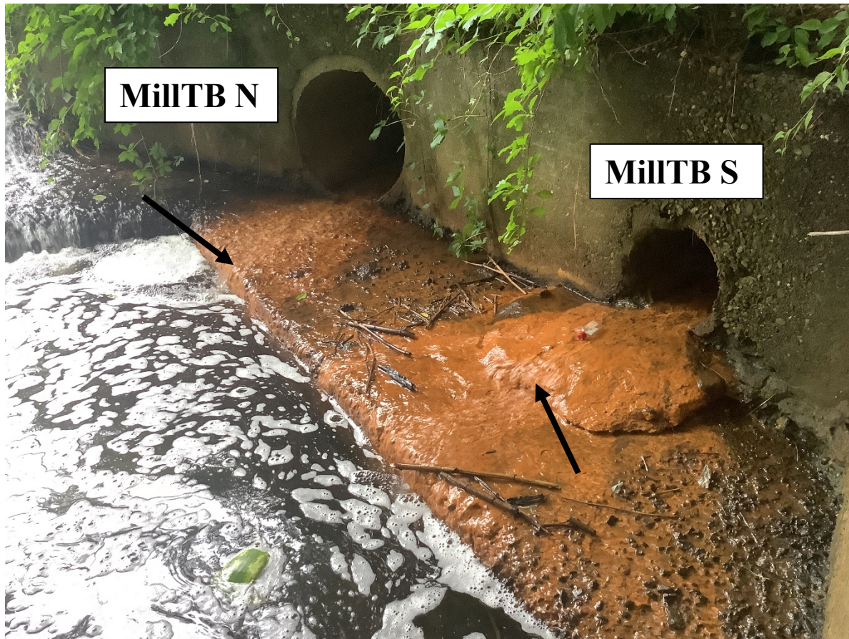
MillTB N&S: Outfalls located on the northern bank of Tatnuck Brook downstream of the Mill Street bridge. Sample collection points indicated by black arrows.
