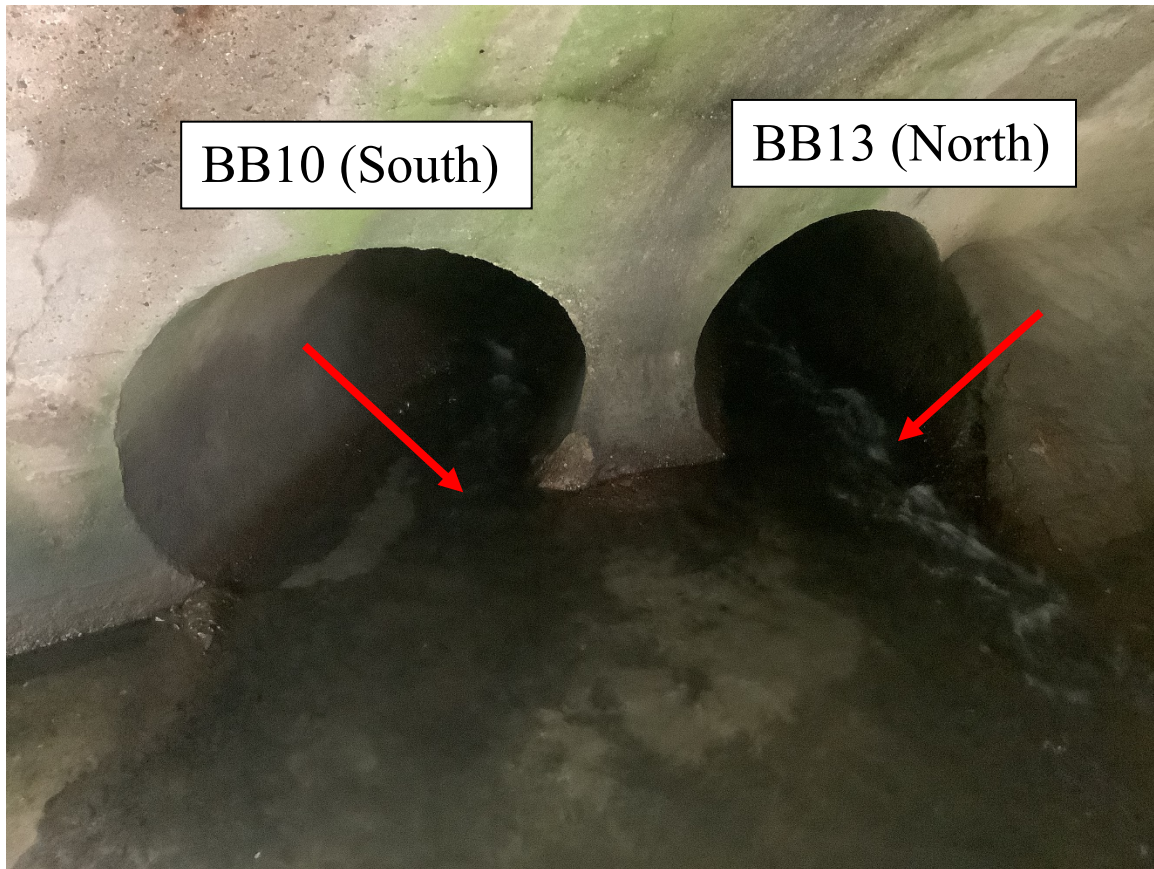
BB10 & BB13: Outfalls located under the bridge at the intersection of Beaver Brook Parkway to the southeast. Sample collection points indicated by red arrows.
