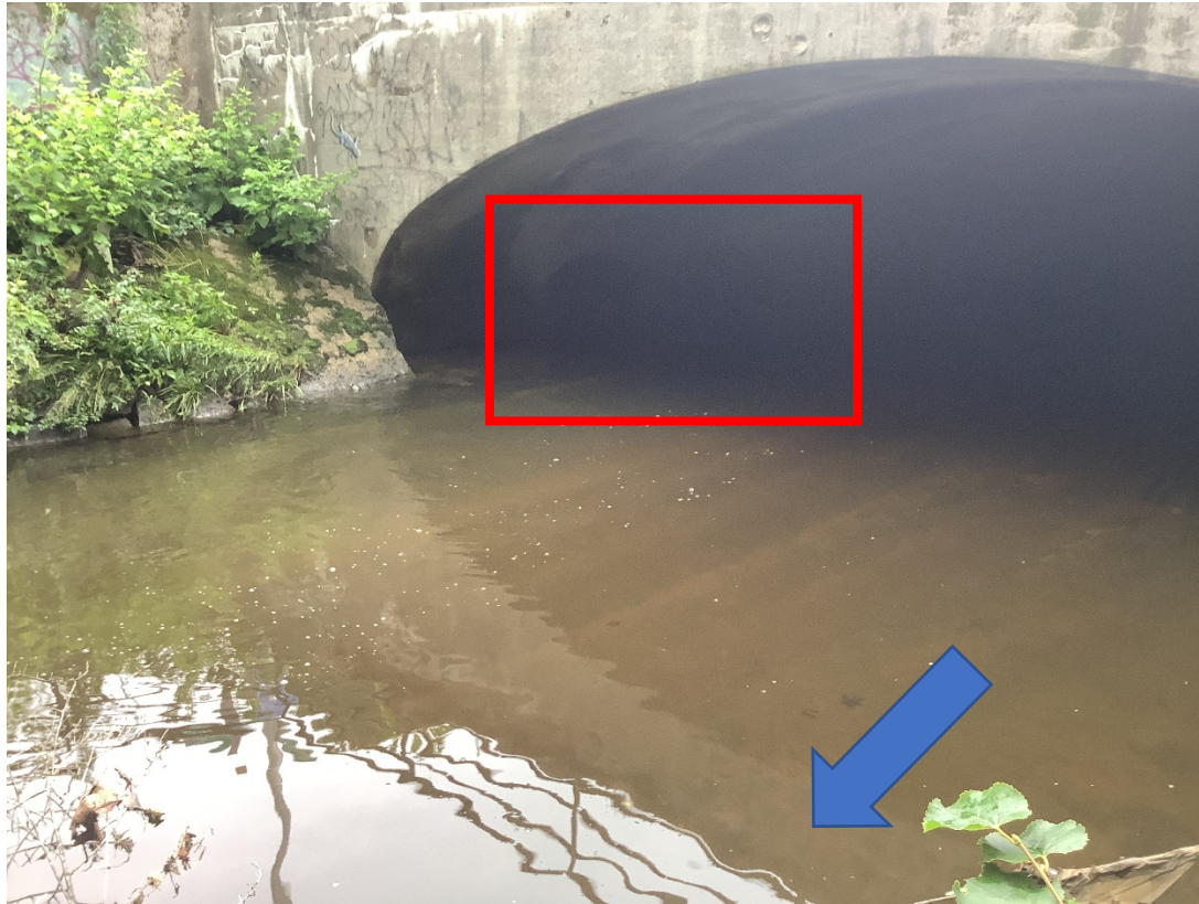
BB10 Down: Outfalls located at the intersection of Beaver Brook Parkway to the southeast. Outfalls are located under the bridge, indicated by a red box. Beaver Brook flow direction indicated by a blue arrow.
