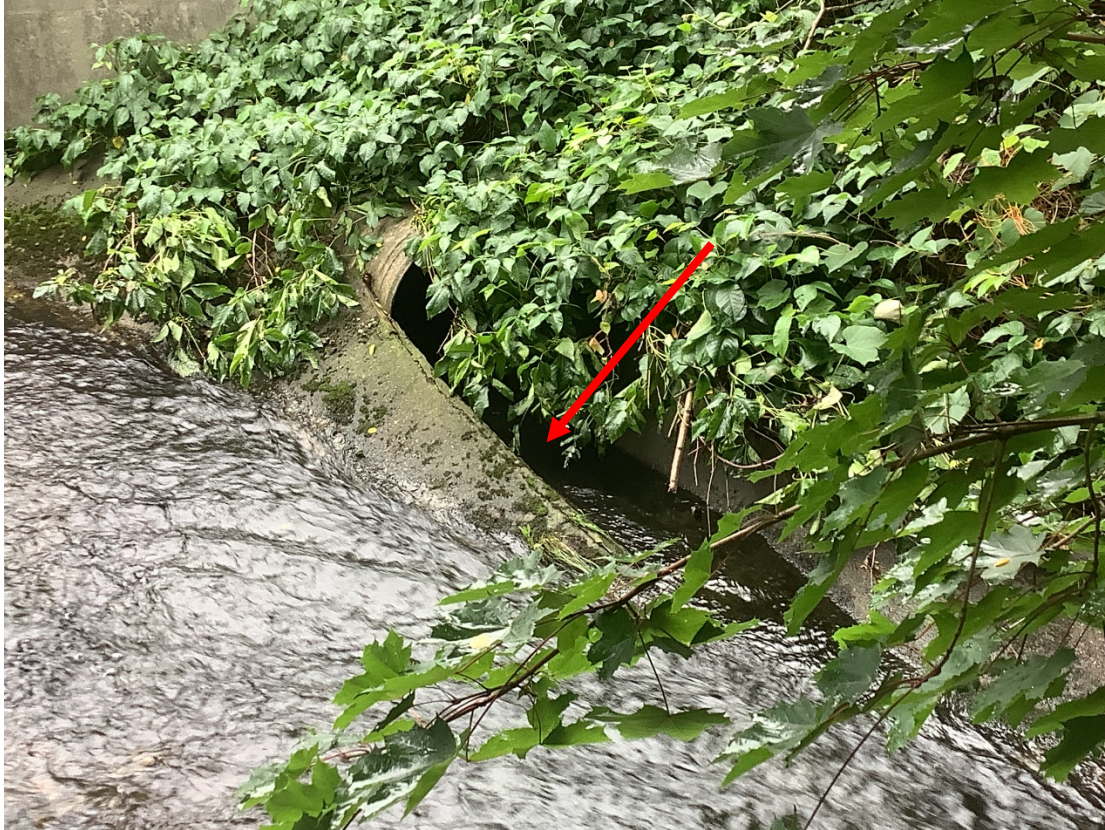
AB07 (2): Outfall located adjacent to the residential property at 116 Holden Street. Sample collection point indicated by a red arrow.
