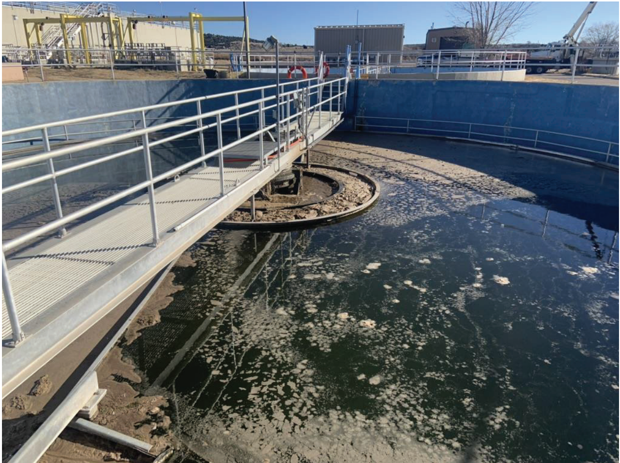
View of the City of Las Vegas WWTF
