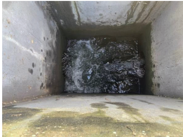
Photo 2: Discharge from west (left) and east (right) clarifiers
