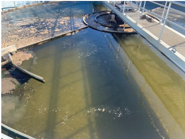
Photo 1: East 2° Clarifier (note sludge blanket level)
