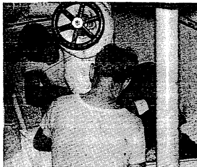
FWT Wm. Katros and Oiler James O'Donnell (background) replace 3rd stage heater trap after renewing 2 eroded sections of pipe.
