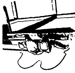
To guard against rust and corrosion all exposed metal surfaces should be given a protective coating that weathers well.
