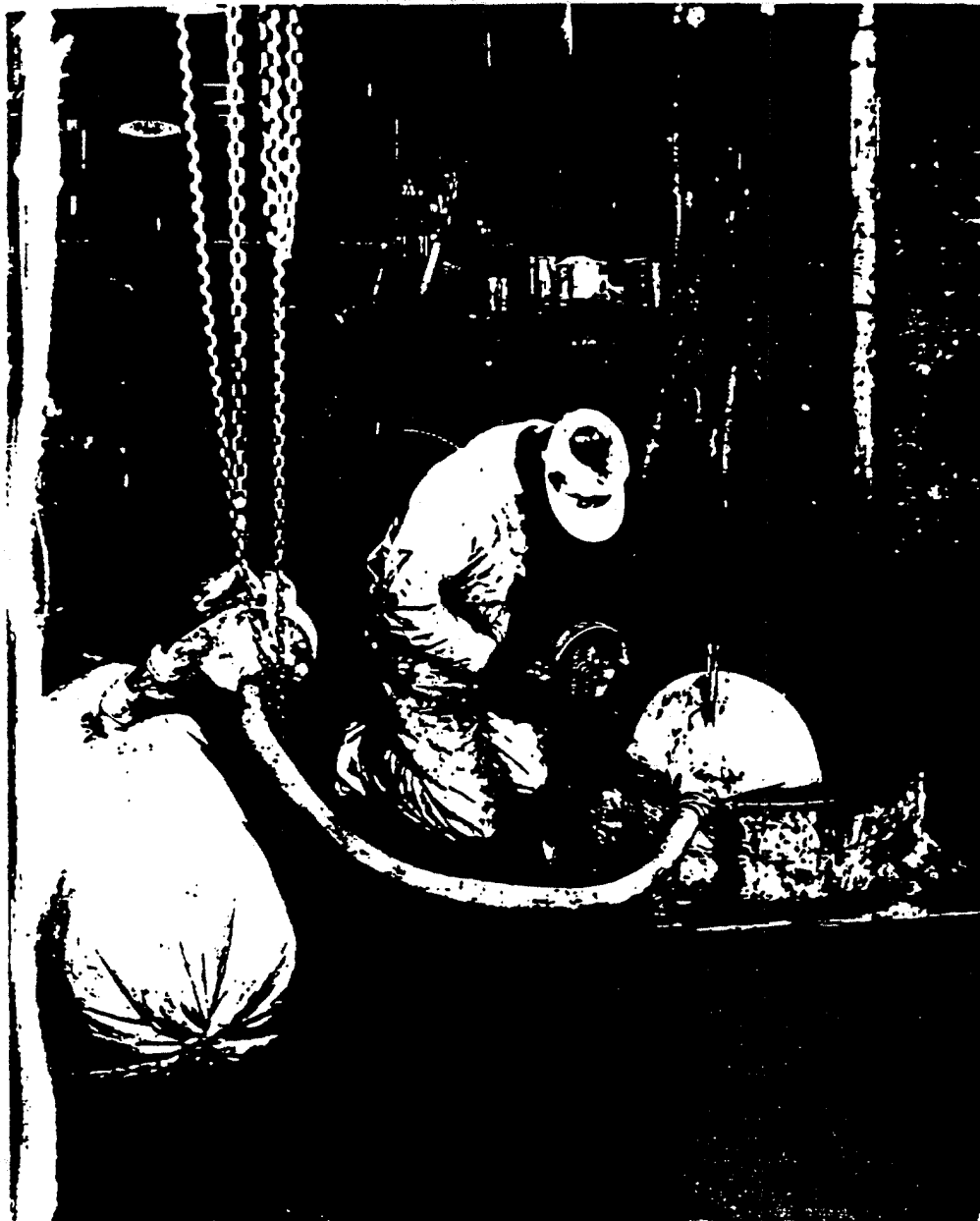
Stone Dressing. This Operation Involves The Creation of Silica Dust. The Makeshift Protective Equipment Here Shown is Inadequate. Potential Danger Associated with this Operation Depends Upon the Quantity of Silica Dust Produced and the Frequency with Which This Operation is Carried Out. Lead Dust At Times May be Created.
