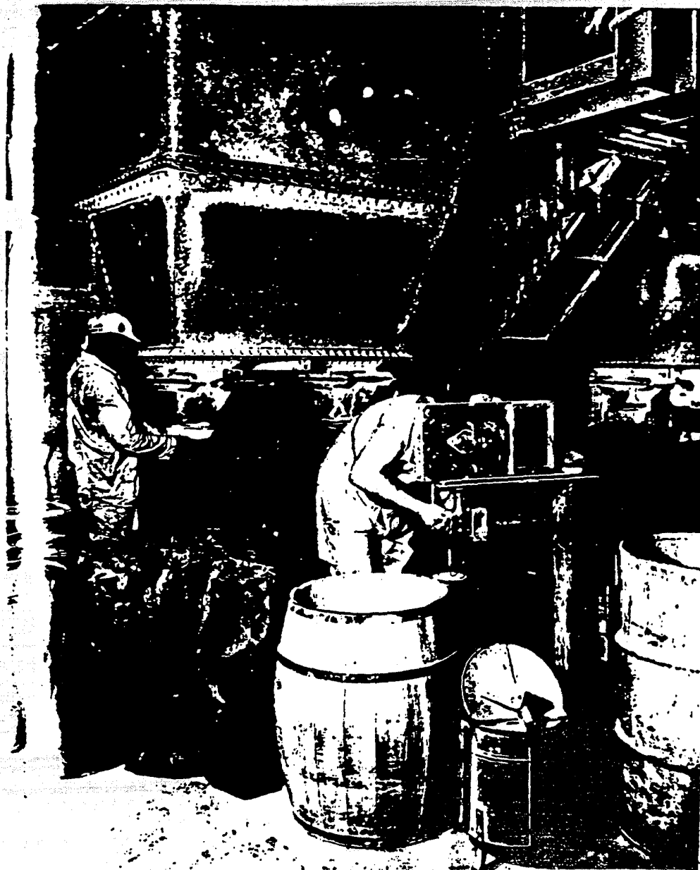
Lithopone Bagging. Lithopone is Essentially Non-Toxic but Grossly Excessive Dust Exposures are Undesirable. The Operation Here Portrayed Calls for Improvement
