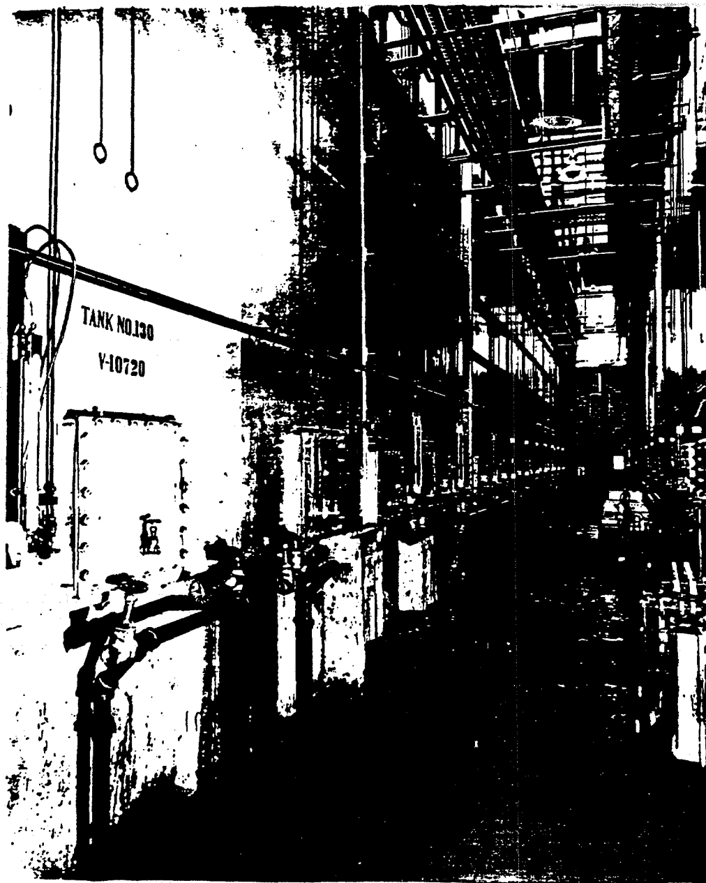
Varnish Storage. The Entry of Workmen Into Storage Tanks is Always Dangerous, Calling For Special Precautions. Insofar as Possible, all Tanks Should be Equipped with Carbon Dioxide Blankets in Order to Avoid the Necessity of Frequent Clean Out Operations
