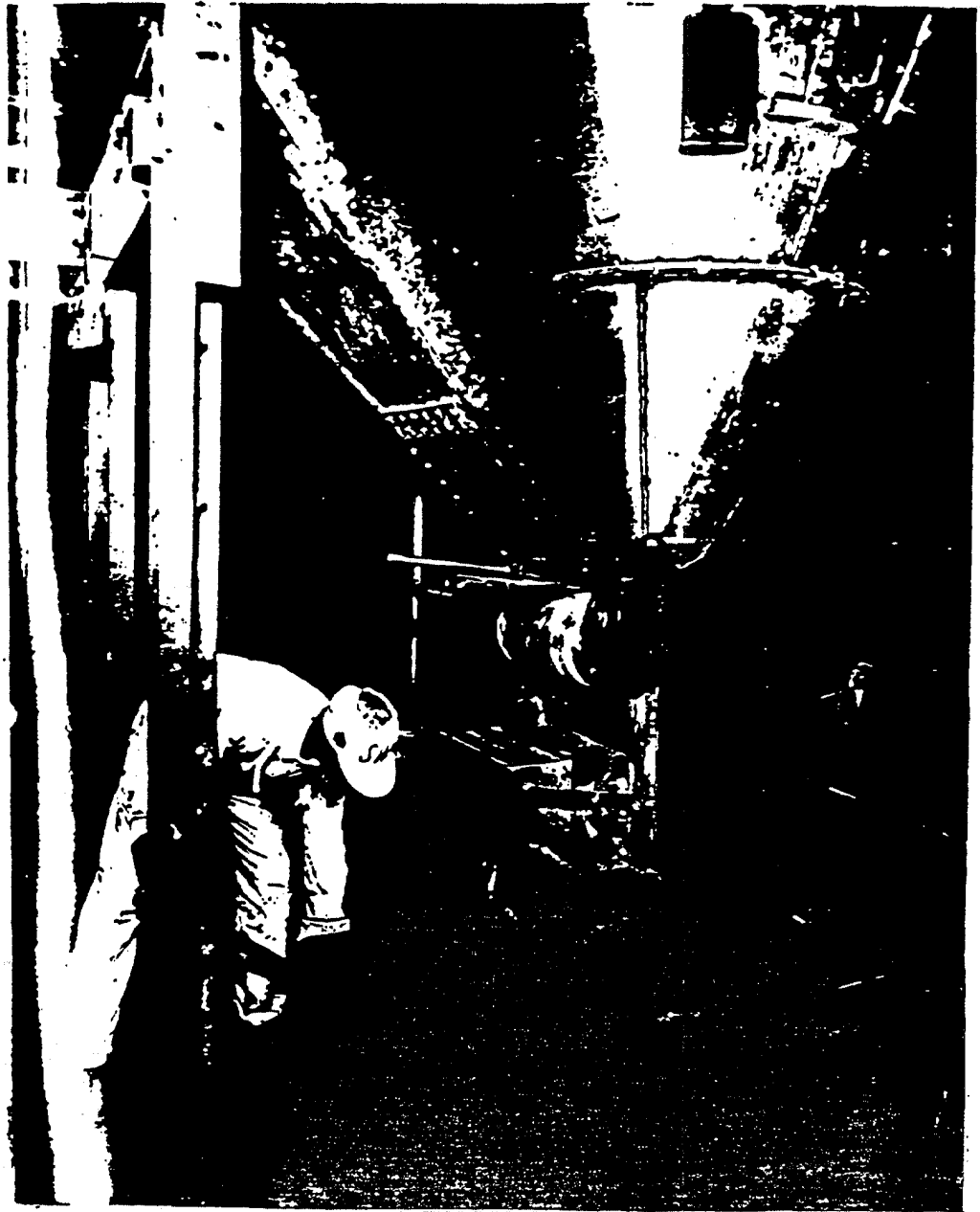
Litharge Milling. Highly Dusty Operation. In the Absence of Consistent Wearing of Respirators, Distinct Exposures May Arise
